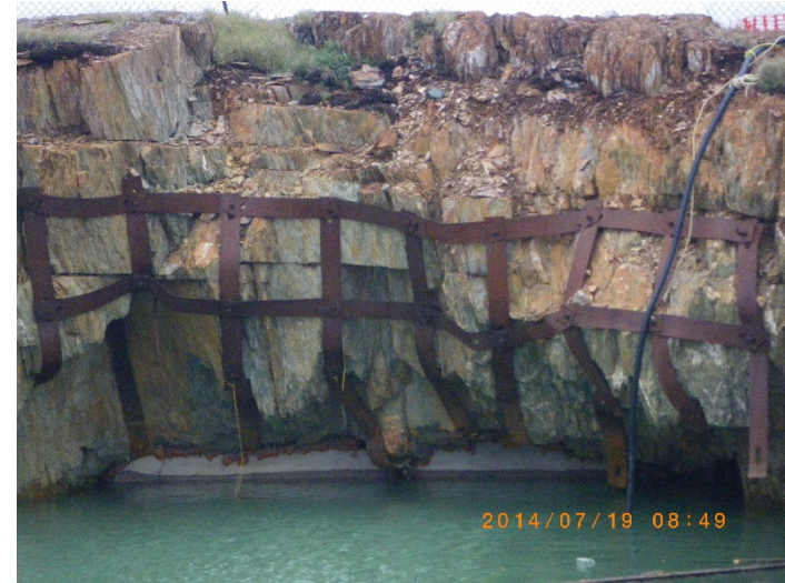
Condition of the reinforcement over the Portal entrance
