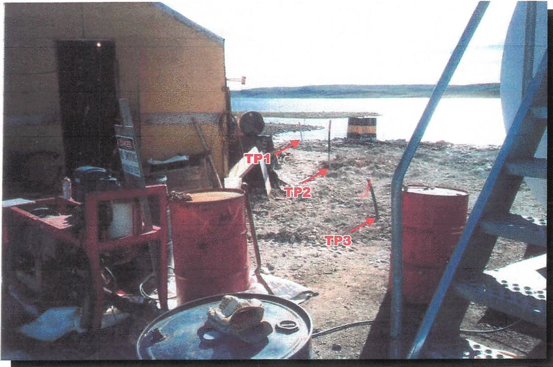
Photo 1 Photograph of test pit/monitoring well locations west of the maintenance shop.
