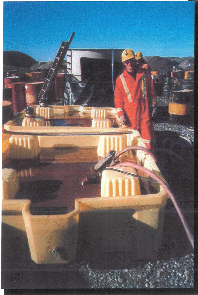
Photo 19 Storage basins for de-emulsification of pre-treatment liquid.
