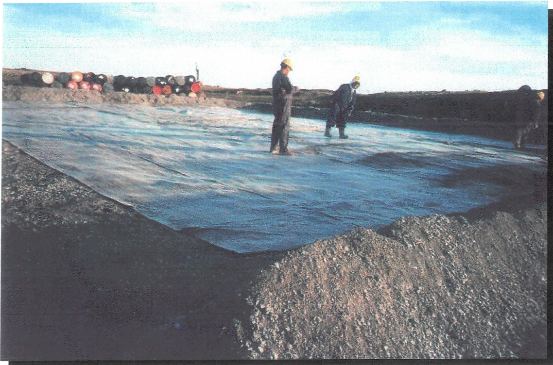
Photo 13 Photograph of Bentomax™ liner used as a protective barrier for landfarm. Looking south.
