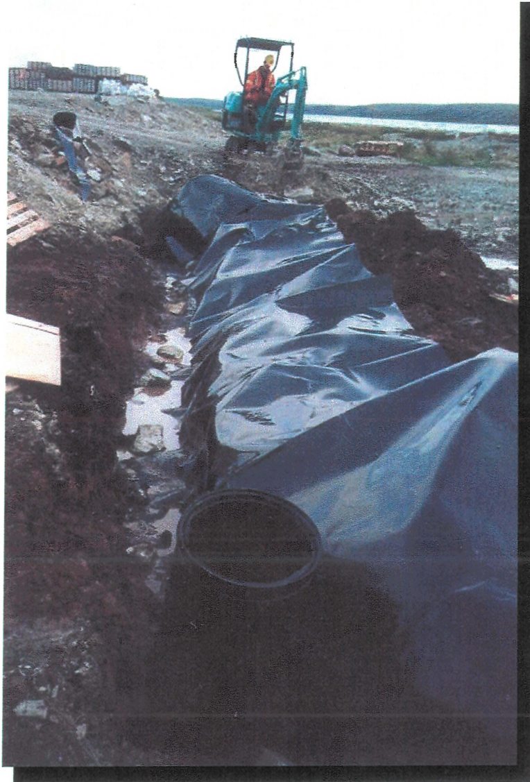
Photo 16 Construction of helipad interception trench.
