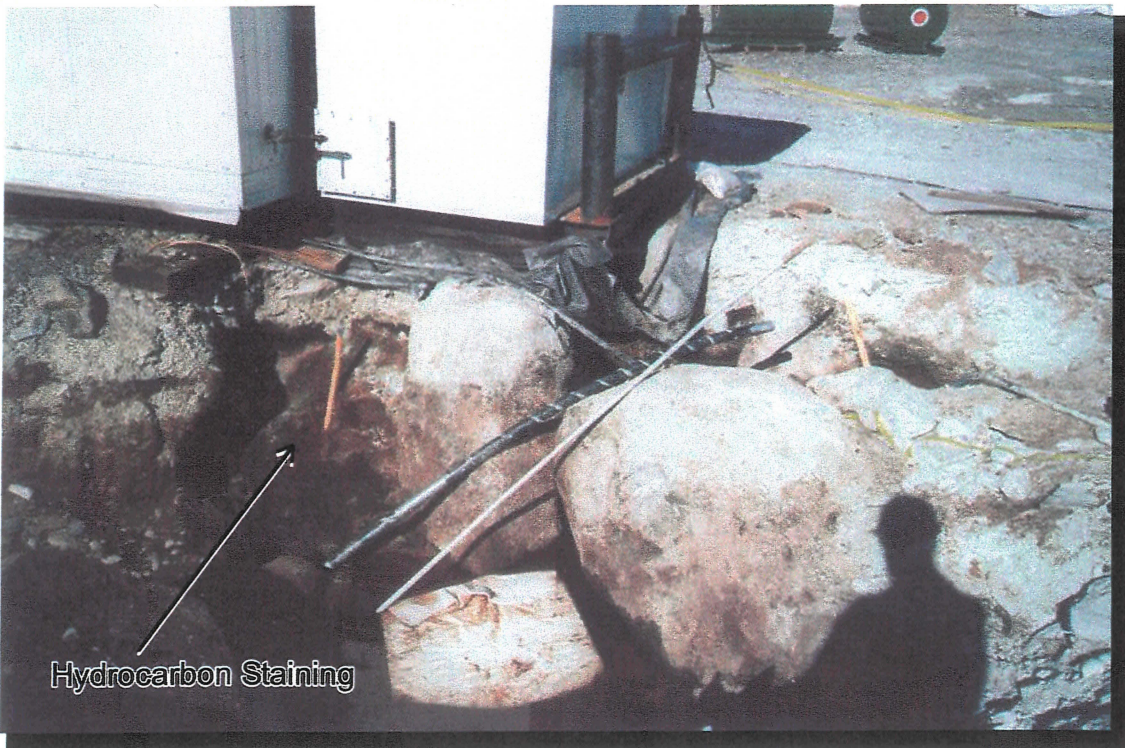
Photo 21 North wall of excavation.
