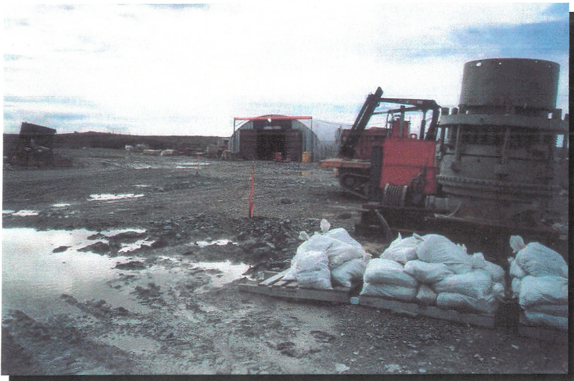
Photo 2 Photograph of test pits/monitoring wells in pad area. Looking south.
