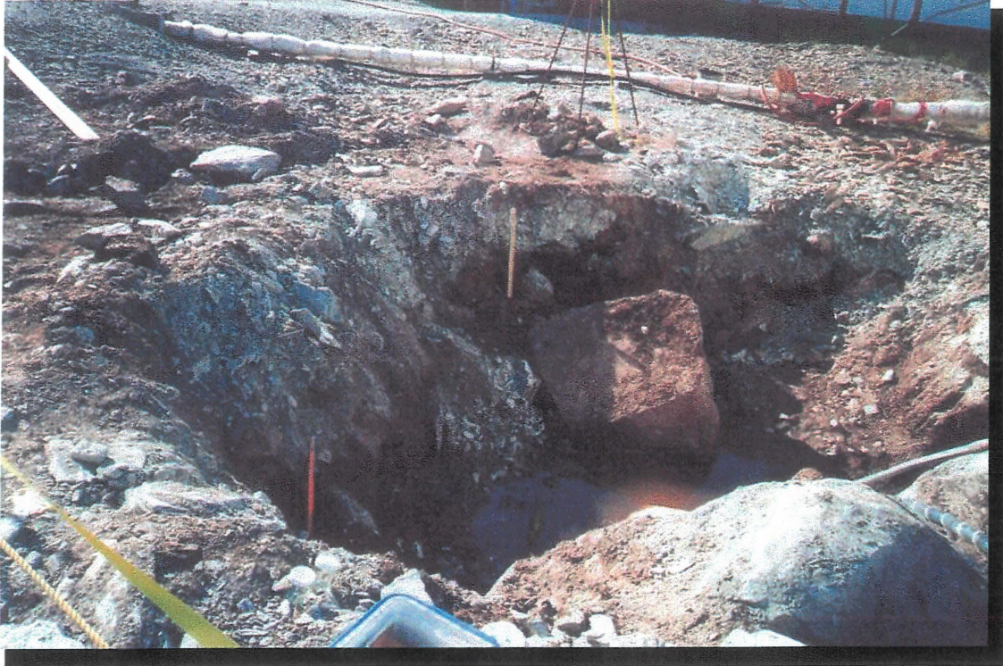
Photo 20 South wall of excavation.
