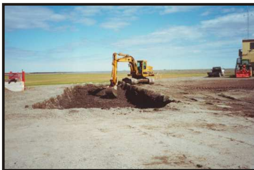
Benzene contaminated soil excavation
