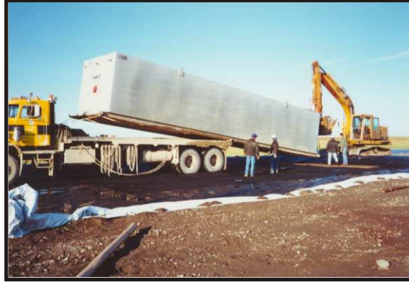
Placement of temporary holding tanks
