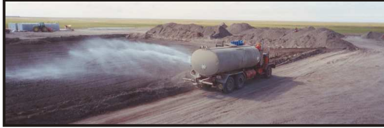
ETEC inoculation of Biocell No. 1
