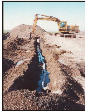
French drain and catch basin construction
