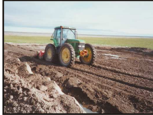
ETEC tractor tilling Biocell No. 3
