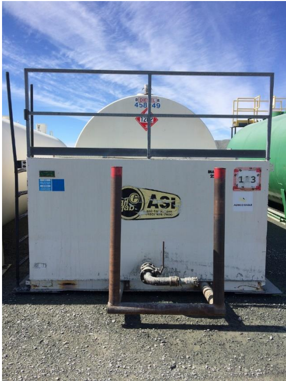
Figure 2, 45,500-liter fuel tank with integrated secondary containment
