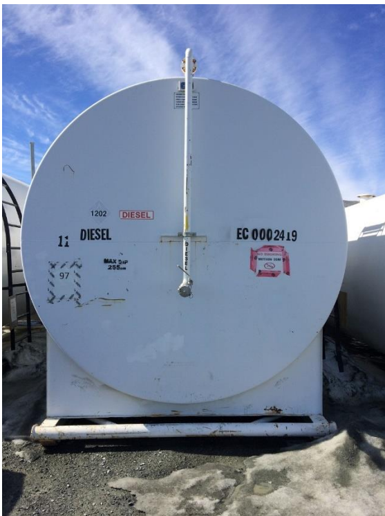
Figure 3, 50,000-liter double wall fuel tank
