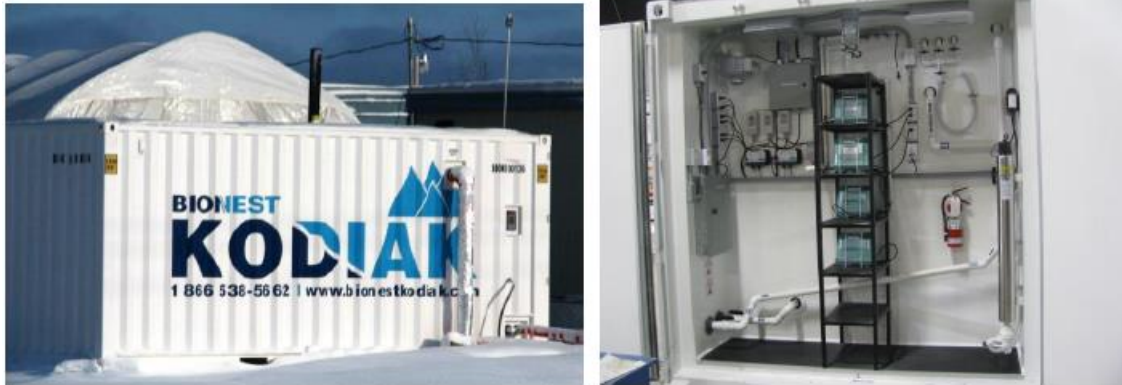
Figure 5, Kodiak Bionest installed in a transport container
