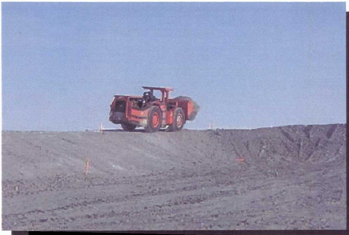
Photo 8 JS250 Scoop with bucket full of material compacting 40 mm Crush along north berm.
