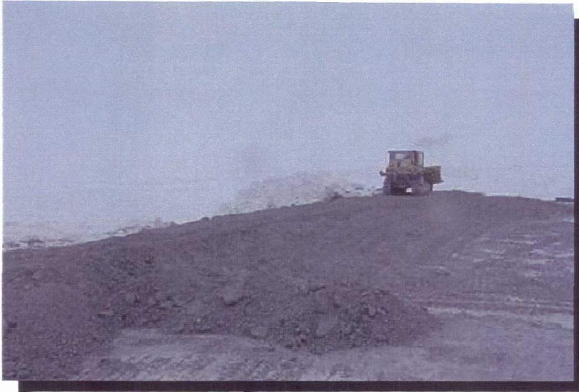
Photo 7 D5H Dozer spreading 40 mm Crush along north berm.
