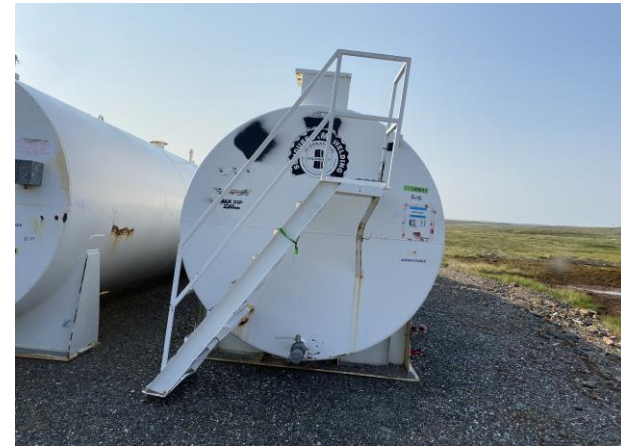
Stairs and bent support arm
