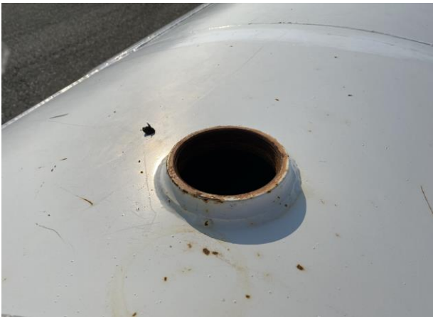
Missing 4" threaded cap
