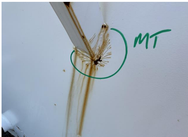
Paint cracked around support arm
