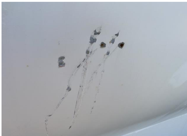
External coating is chipped
