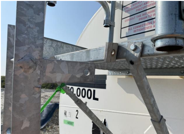
Not properly connected
