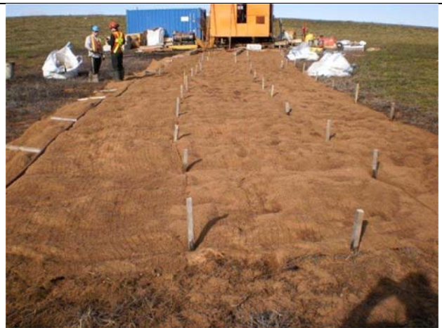
July 14, 2011. View west looking at the Orbit 25 drill rig. Coconut matting placed to provide temporary insulation for the bare ground while a restoration plan is developed.
