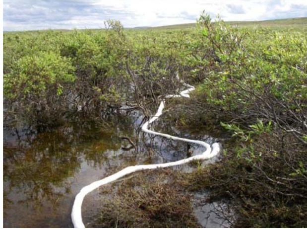
July 14, 2011. View south along Stickleback Outflow (inflow to Aimaokatalok Lake). Booms placed to absorb hydrocarbons in the event that any residuals drain into the water downhill of the Orbit 25 Drill Rig.
