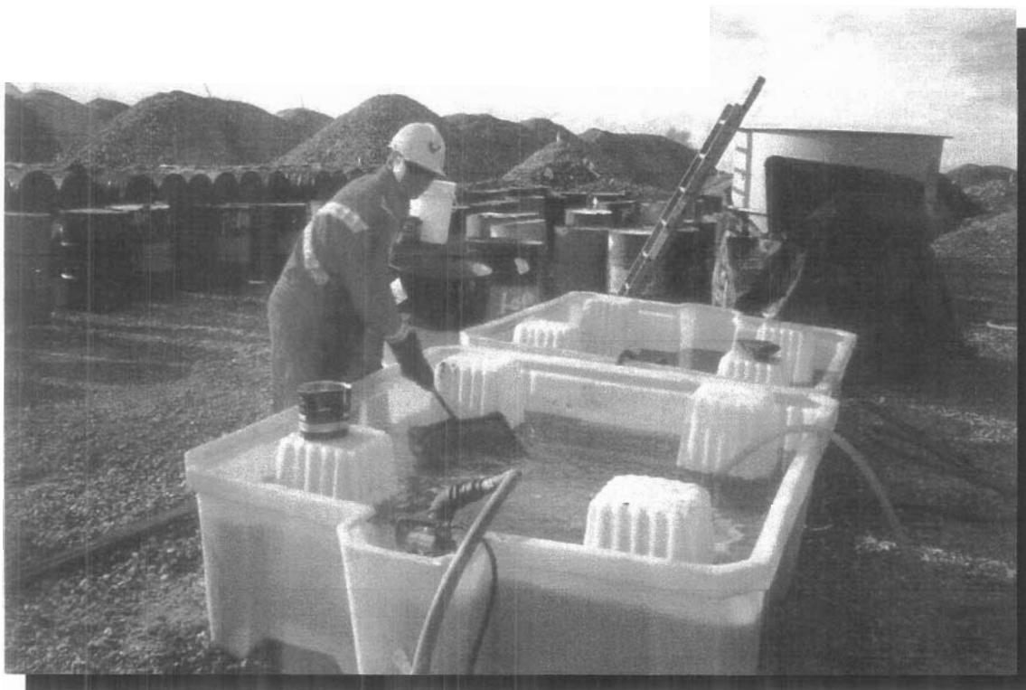
Photo 23 Removal of floating material with screen filter.
