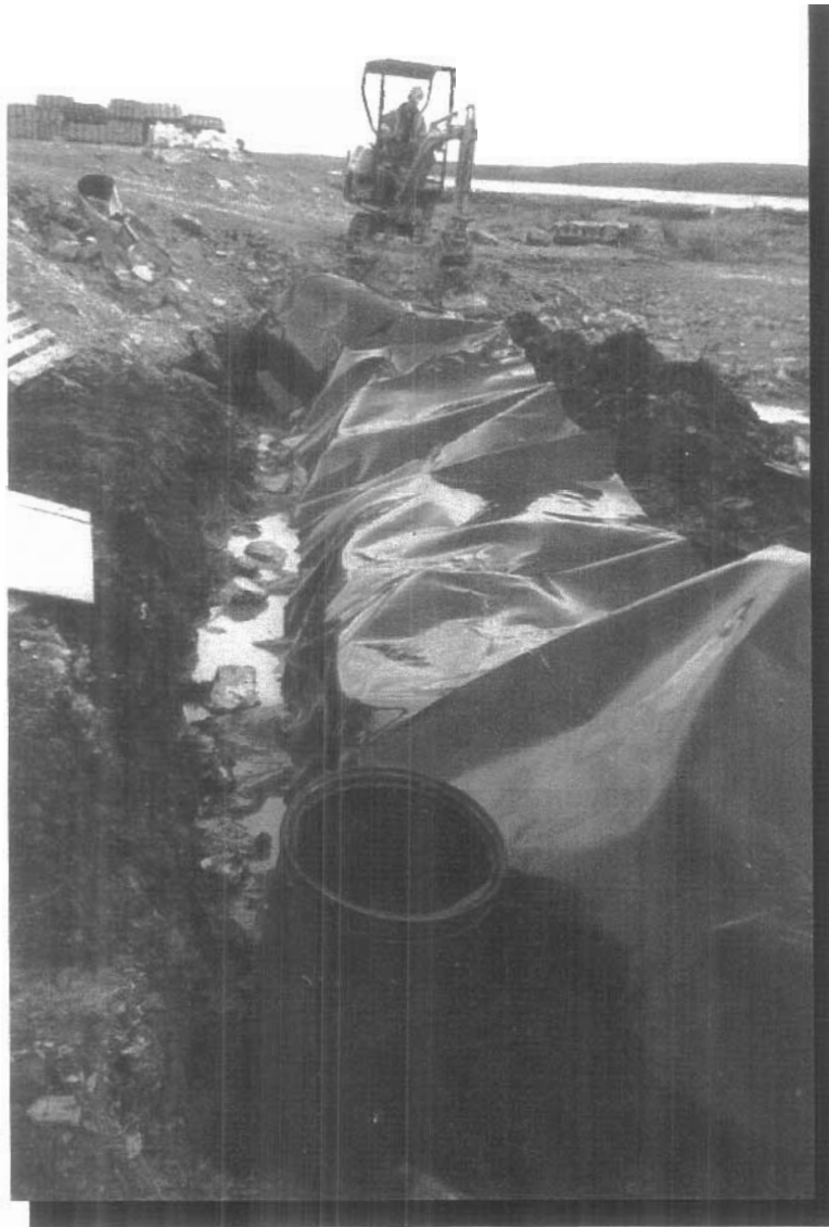
Photo 10 Construction of helipad interception trench.
