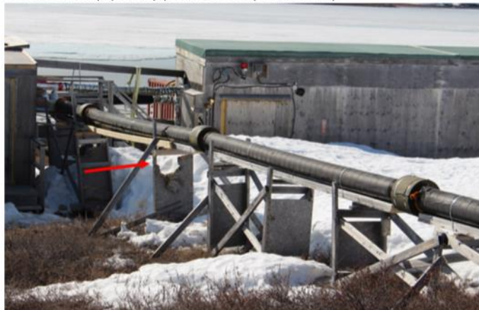
Figure 1. Pipeline and pipe connection of main kitchen grey water line
