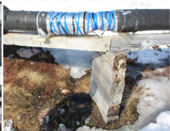
Figure 1. Pipeline and pipe connection of main kitchen grey water line
