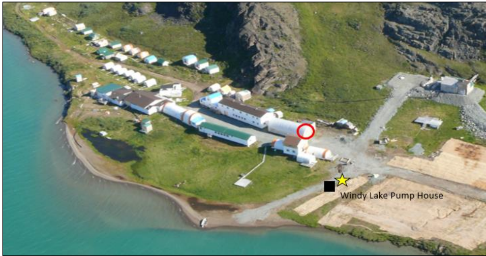
Plate B.1. Windy Camp (Note: Red circle is fuel storage location, smaller storages locations may vary. Yellow star indicates spill kit location.)
