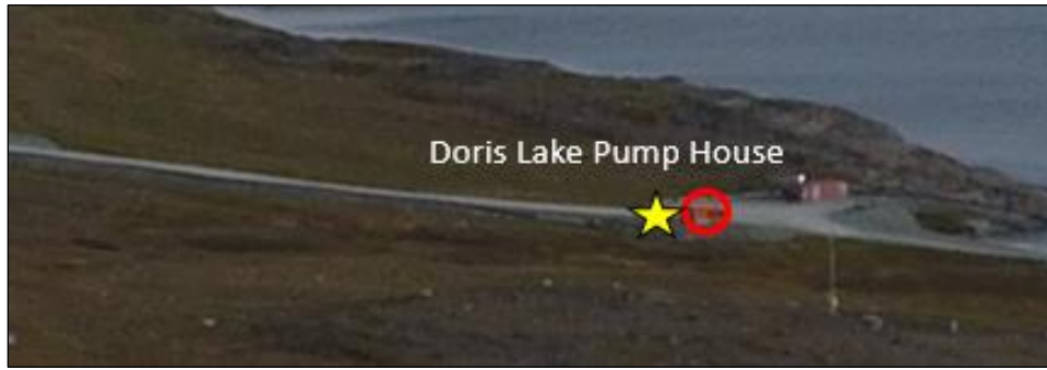
Plate A.3. Doris Lake Freshwater Pumphouse (Note: Red circles are fuel or chemical storage locations, smaller containment locations may vary. Yellow stars indicate default spill kit locations.)
