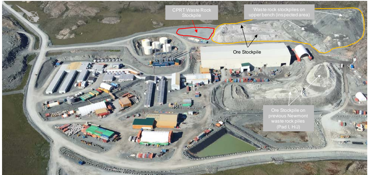
Figure 1-1: Waste Rock and Ore Stockpile Locations, Doris Mine (Photo taken August 5, 2018)
