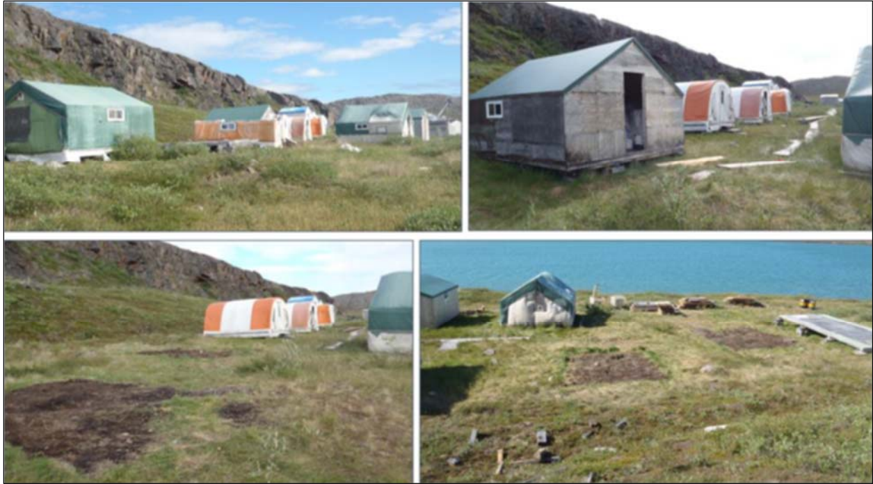
Photo 13.1-2. Cabin and tent structures prior to reclamation (top) and post reclamation (bottom). Waste piled and segregated for transport to Doris Waste Management Facility shown in background.
