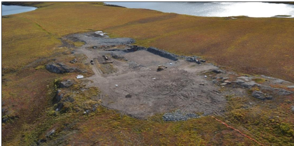
Plate B.2. Patch Laydown Facility (Note: Red circle is fuel storage location, smaller storages locations may vary. Yellow star indicates spill kit location.)
