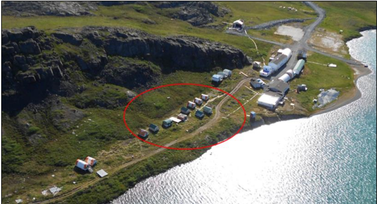
Photo 13.1-1. Windy Camp pictured in 2013. Area of 2018 reclamation activities denoted by red circle.
