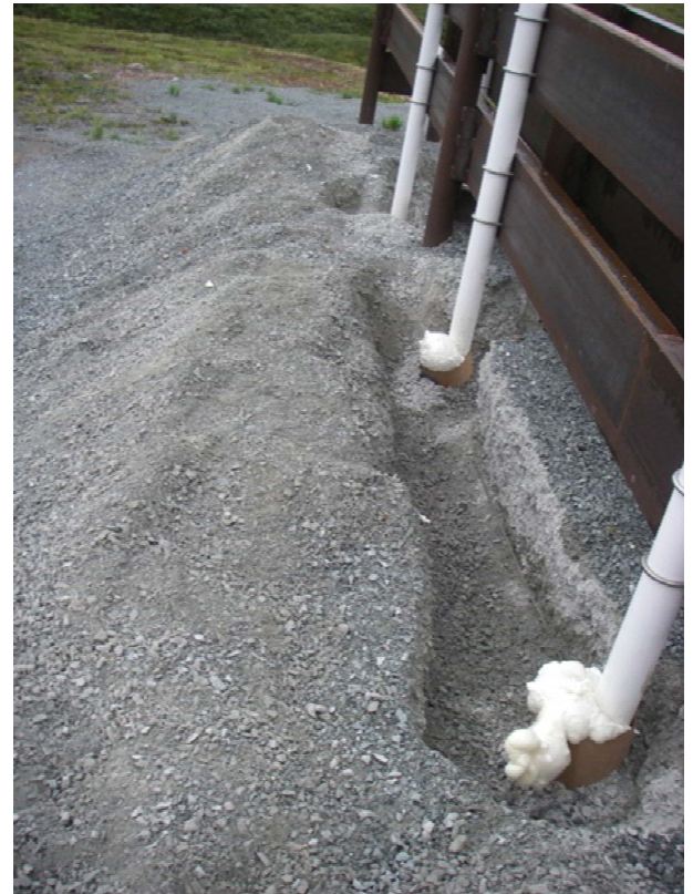
Thermosyphon status thermistors after being heat-insulated using expanding spray foam.
