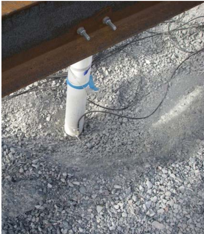
Thermosyphon status thermistors attached to thermosyphon risers using epoxy resin and zip-ties.
