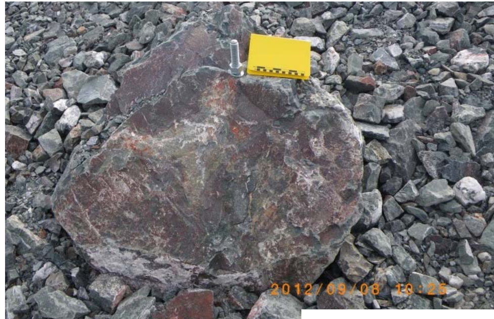
Examples of crest survey monument. Note the small rock bolt /anchor installed in the boulders seated into the dam shell.
