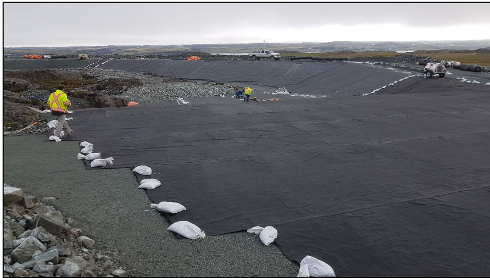
Geotextile placement 0+000 to 0+100. July 8, 2019
