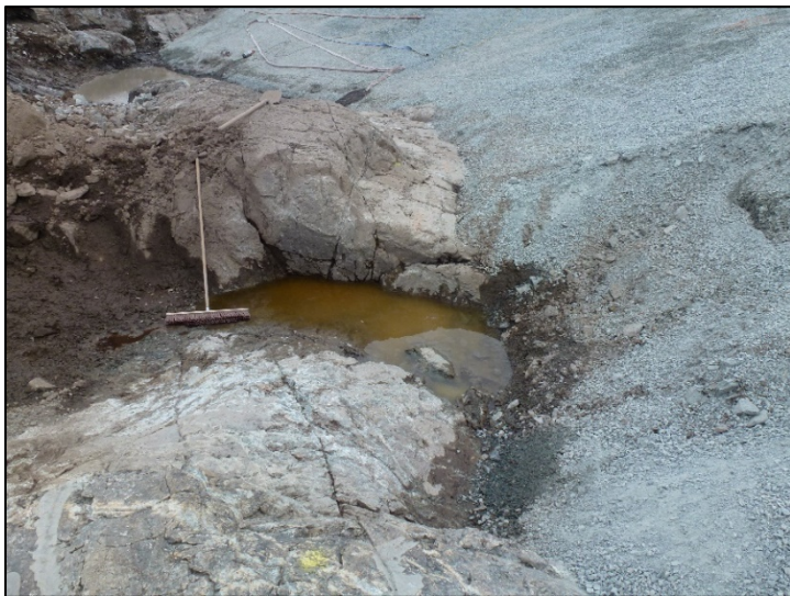
Cleaning of bedrock at liner tie-in or plinth contact 0+100 to 0+160. June 26, 2019
