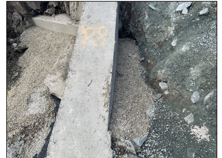
Concrete cast, Sopramastic placed along joints with bentonite crush. July 25, 2019
