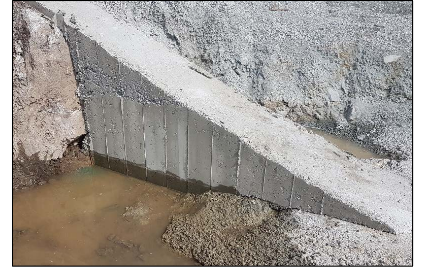
Formwork removed leak testing plinth 8. July 4, 2019
