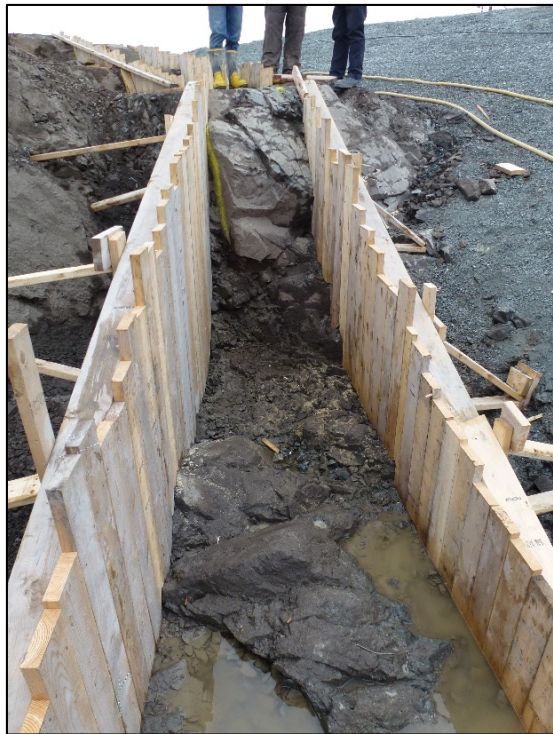
Formwork for plinth 5 contact. June 30, 2019
