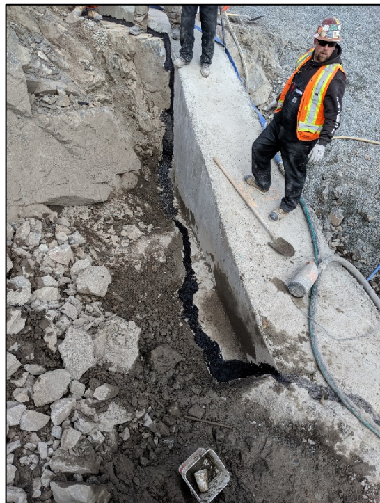
Sikaset Plug and Sopramastic along join July 17, 2019
