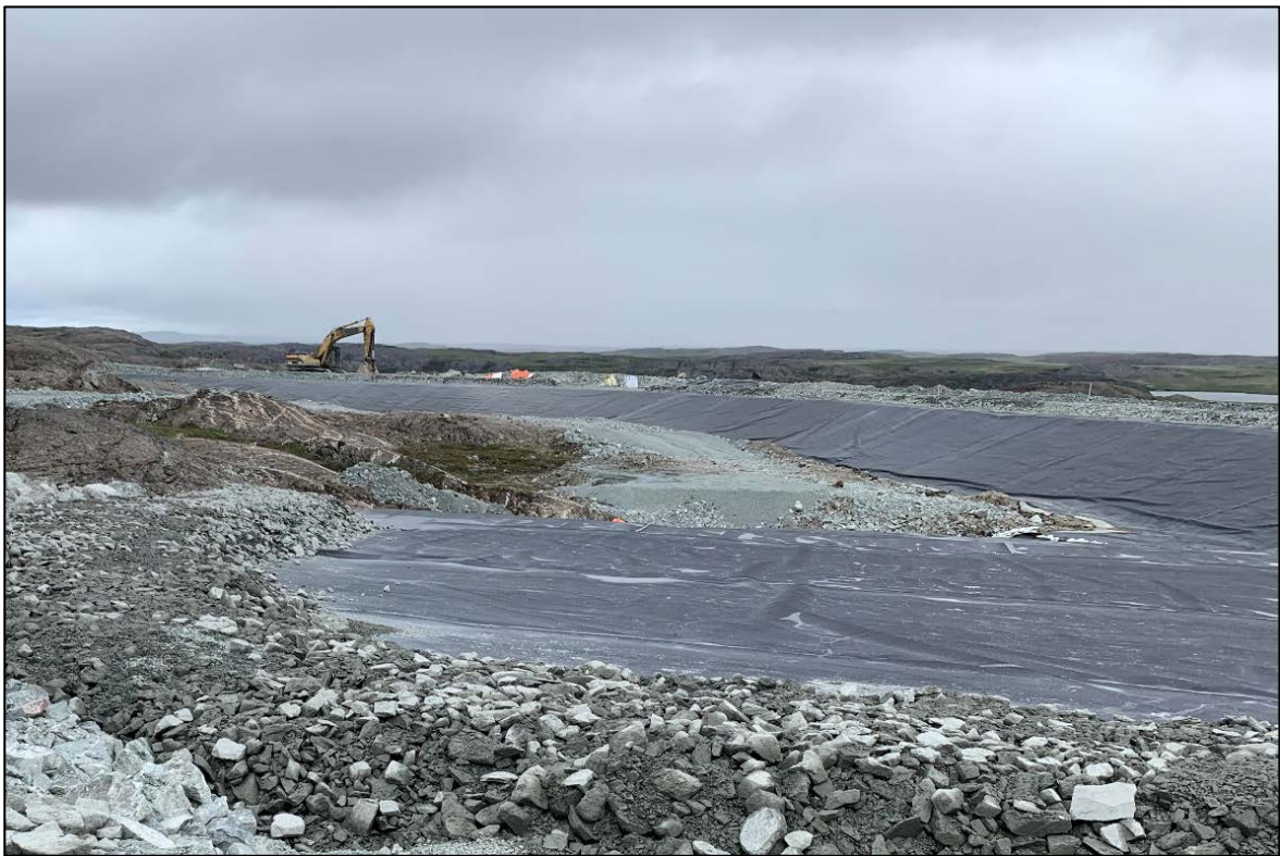
Liner anchor material 0+000 to 0+225. July 28, 2019
