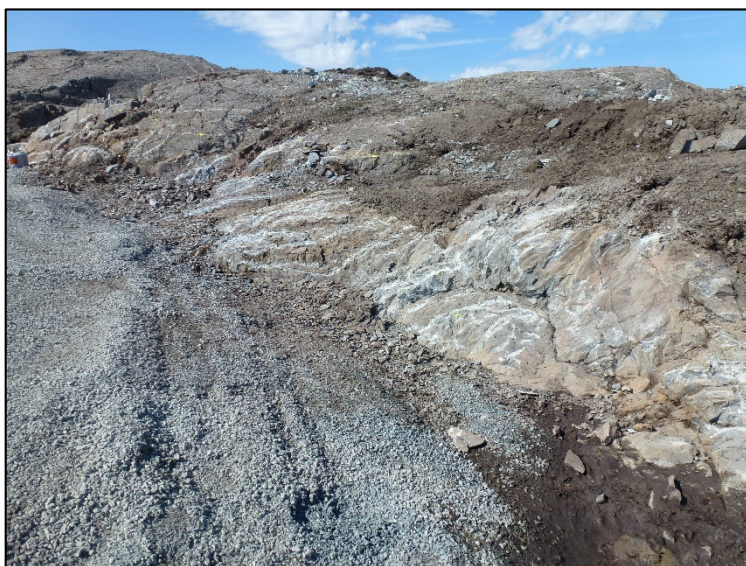
Cleaning of bedrock at liner tie-in or plinth contact 0+050 to 0+100. June 25, 2019
