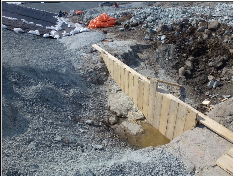
Formwork for plinth contact. June 29, 2019
