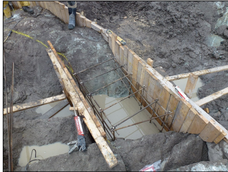
Formwork and steel reinforcing for plinth 3. June 30, 2019
