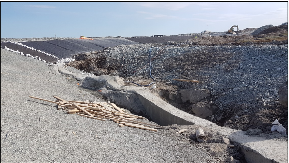
Concrete grouting for liner tie-in 0+160 to 0+225. July 3, 2019
