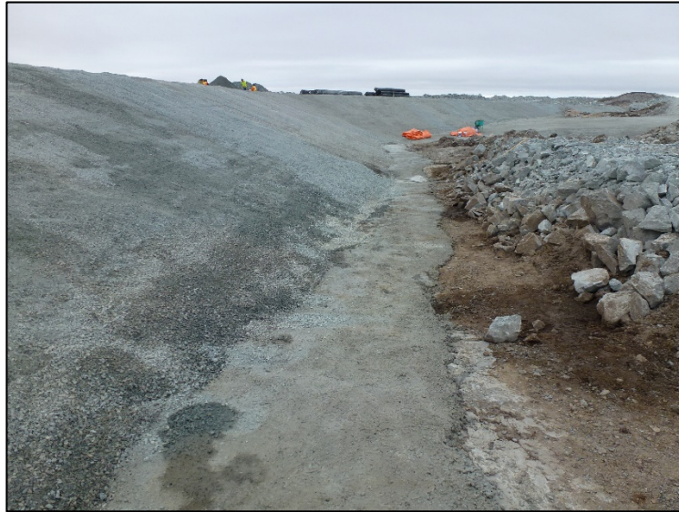
Placement of bedding material 0+000 to 0+160. June 26, 2019
