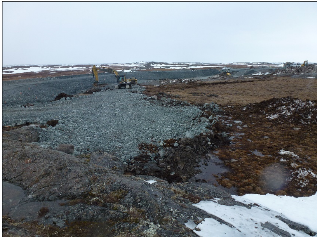
Placement of additional ROQ to fill deeper than expected overburden 0+050 to 0+075. June 15, 2019
