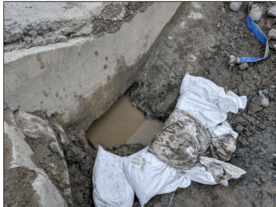
Void cleaned below plinth 3. July 15, 2019
