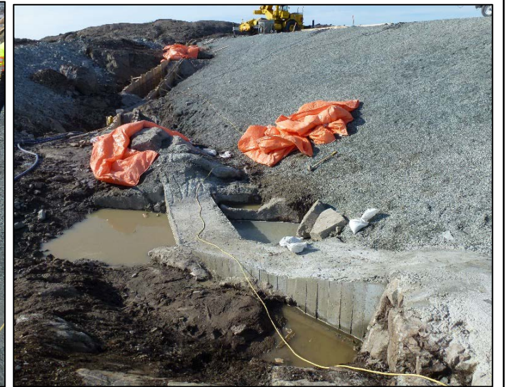
Formwork stripped plinth 2 and plinth 3 July 1, 2019
