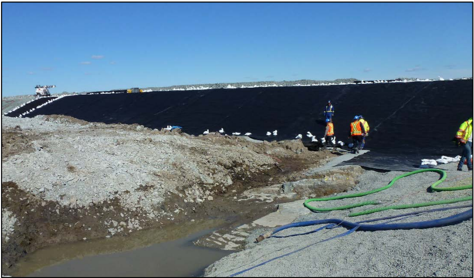
Geotextile and liner placement 0+050 to 0+100. June 28, 2019
