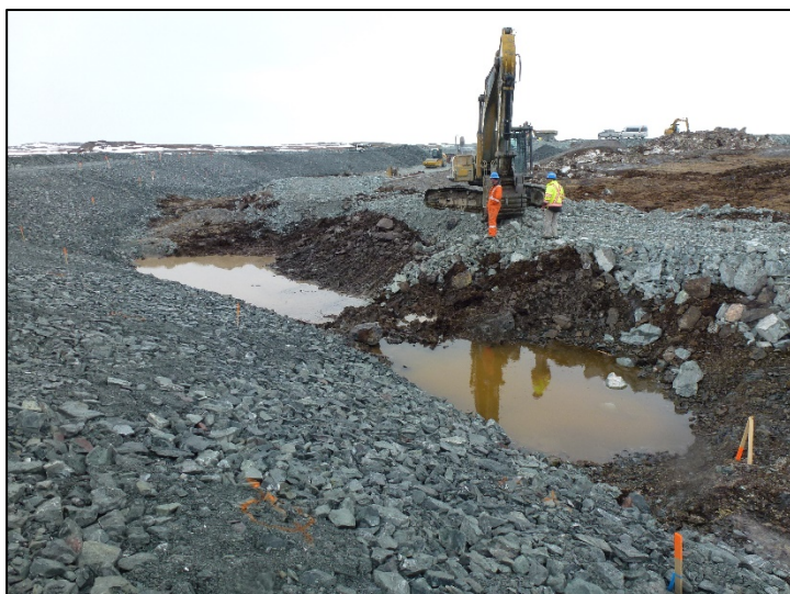
Excavation of overburden at upstream toe to expose Bedrock 0+160 to 0+225. June 15, 2019
