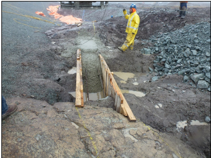
Casting of concrete plinth 7 June 30, 2019
