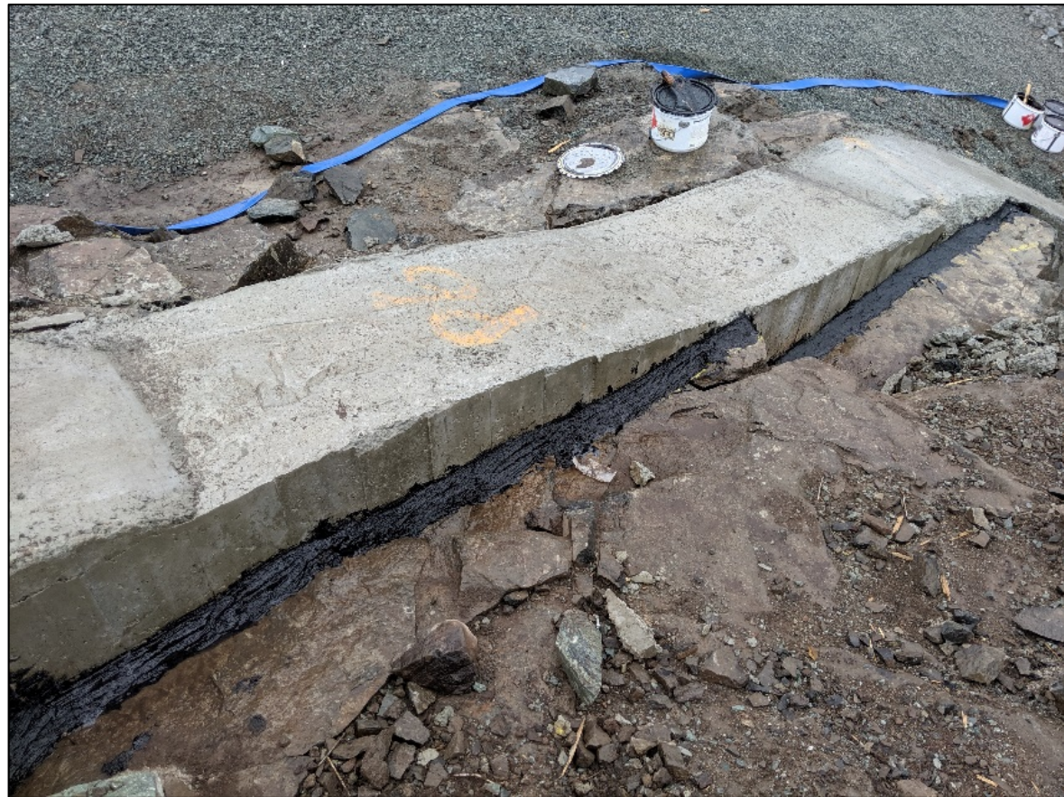
Sopramastic placed for voids plinth 6 July 16, 2019
