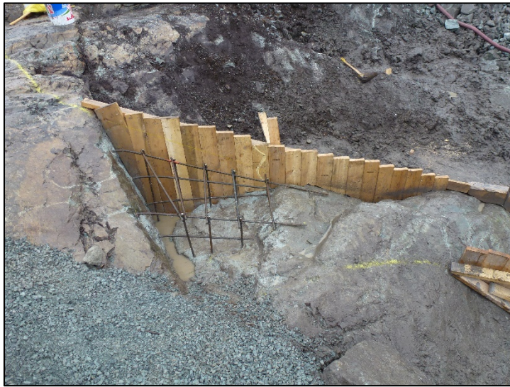
Formwork and reinforcing plinth 2 June 30, 2019
