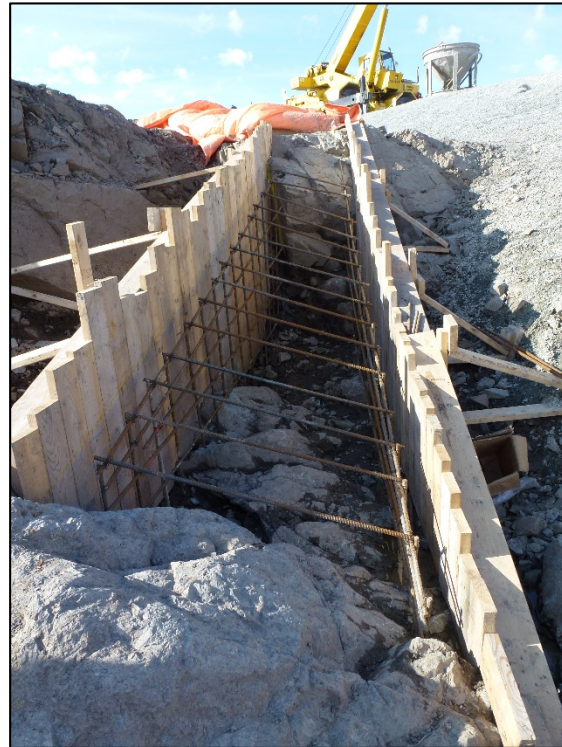
Formwork and reinforcing for plinth 5. July 1, 2019
