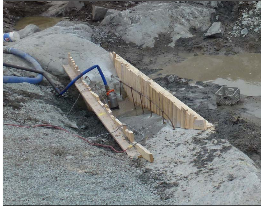
Contact rock cleaned and formwork placed plinth 10. July 2, 2019
