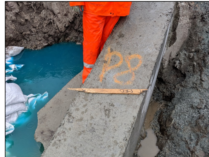
Concrete grout cast, dye test conducted. July 15, 2019
