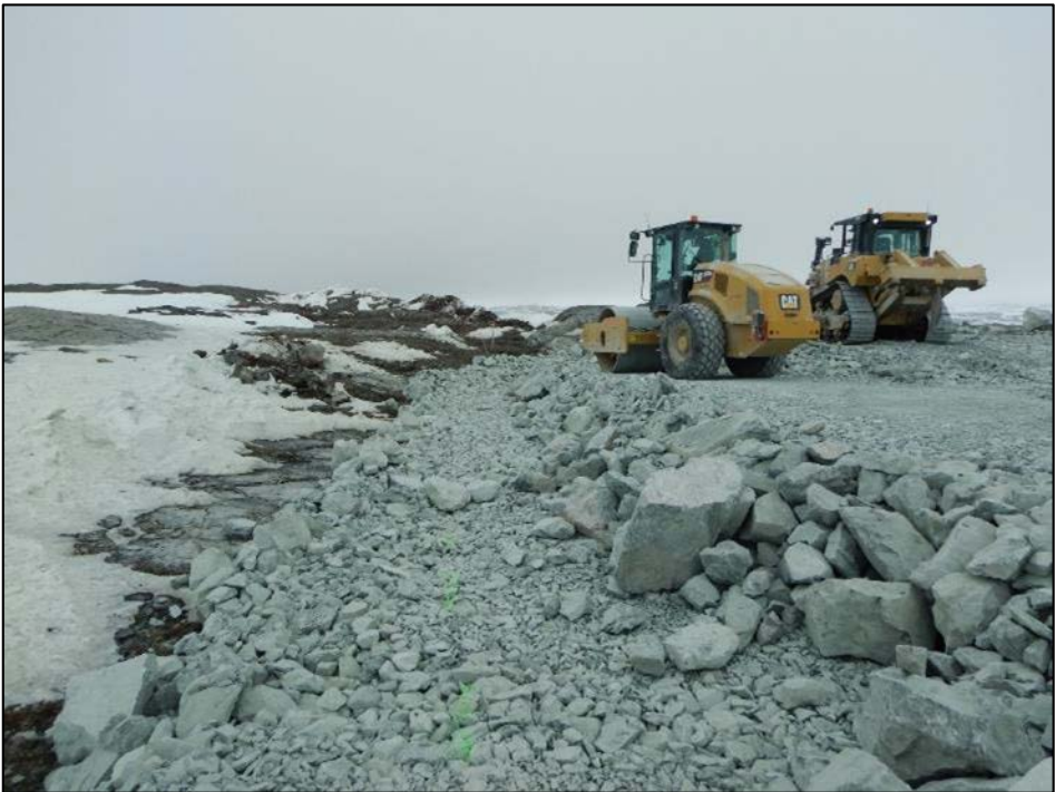
ROQ placement and roller compaction. June 3, 2019
