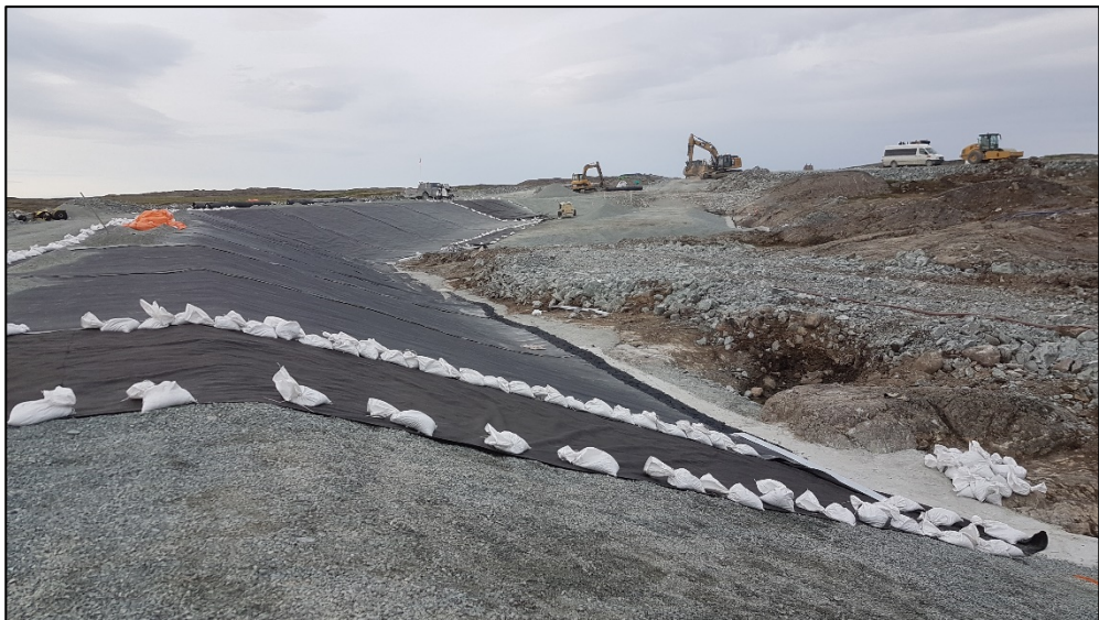
Geotextile and liner placement 0+100 to 0+160. July 6, 2019
