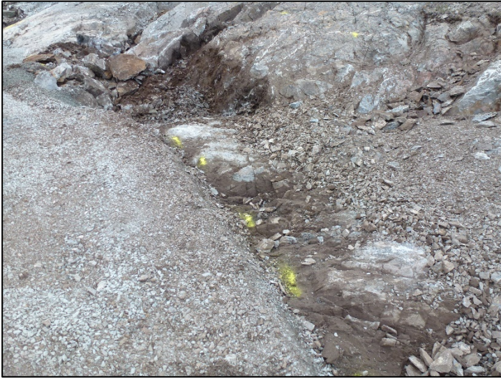
Cleaning of bedrock at liner tie-in or plinth contact 0+000 to 0+050. June 26, 2019
