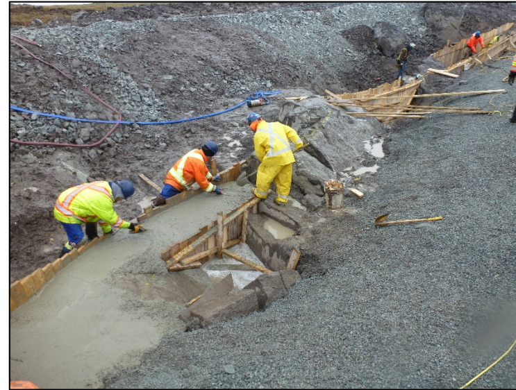
Concrete being floated plinth 2 and plinth 3 June 30, 2019
