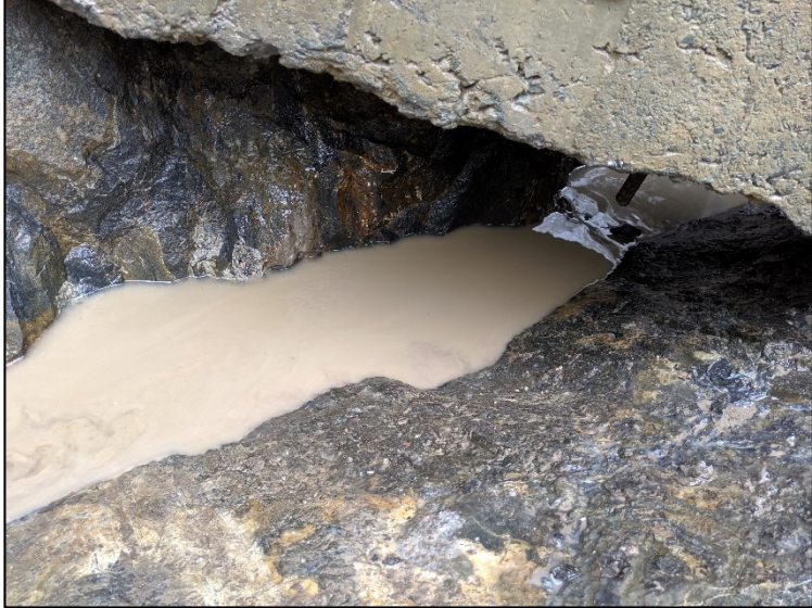
Void cleaned below plinth 4 July 13, 2019
