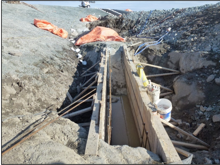
Formwork and reinforcing for plinth 4. July 1, 2019
