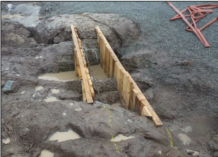
Formwork and steel reinforcing for plinth 7. June 30, 2019
