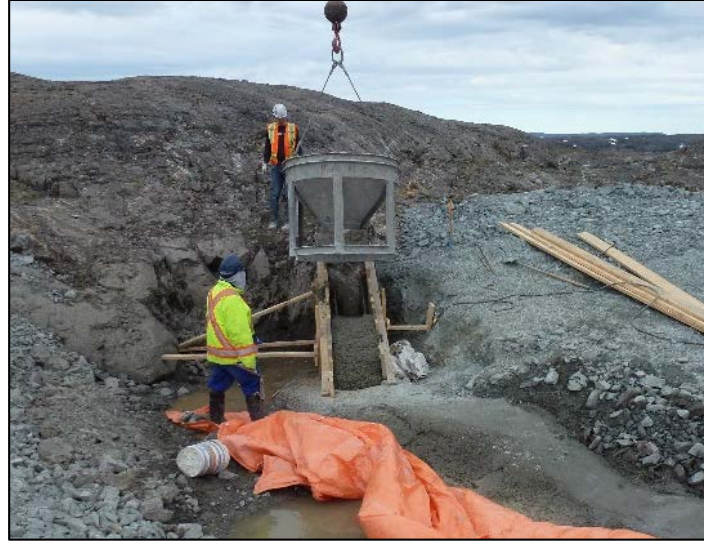
Concrete casting plinth 8 July 2, 2019
