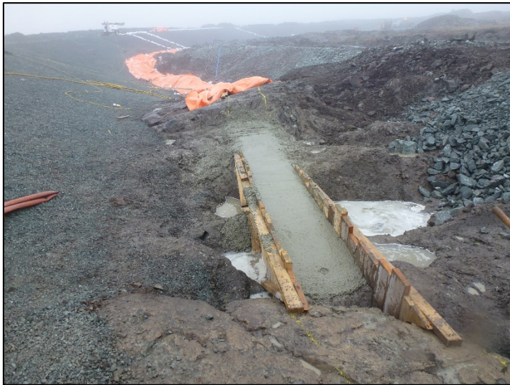
Concrete cast plinth 7 June 30, 2019
