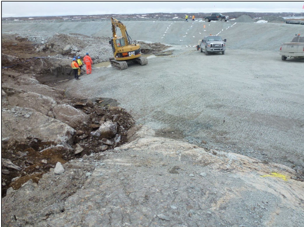
Placement of additional ROQ and bedding material to fill deeper than expected overburden 0+050 to 0+075. June 26, 2019
