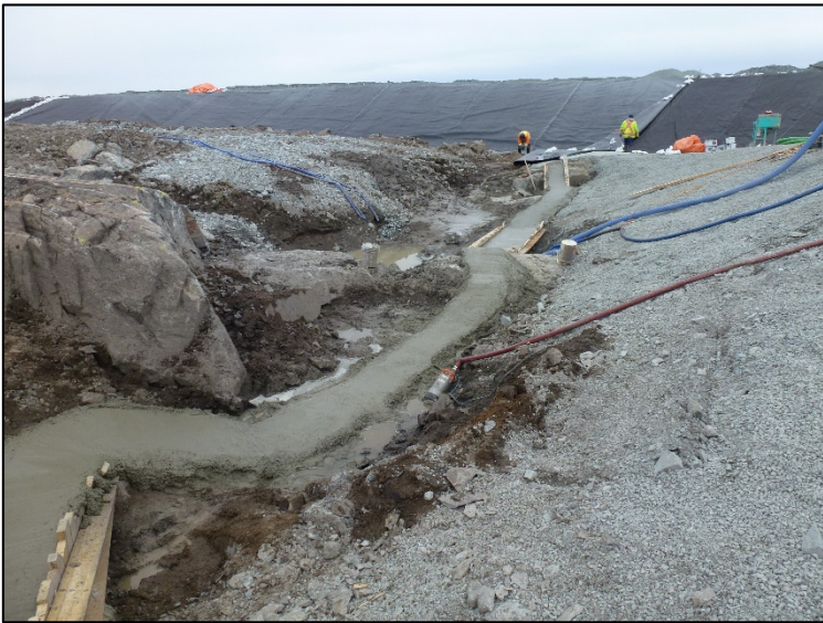
Concrete grouting 0+050 to 0+075. July 2, 2019
