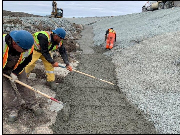
Concrete liner tie-in 0+120 to 0+160. June 24, 2019
