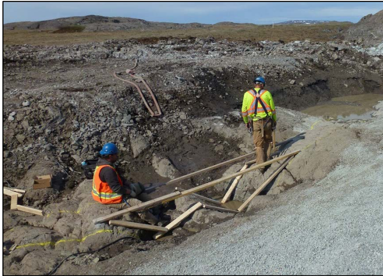
Cleaning and formwork for plinth 7. June 29, 2019
