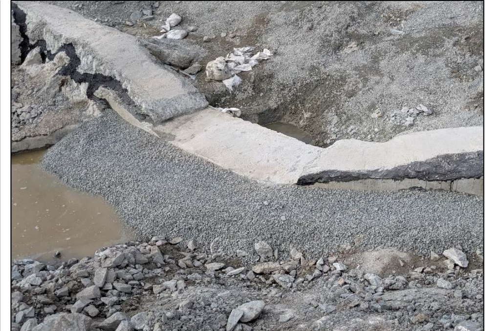
Bentonite crush placed July 17, 2019
