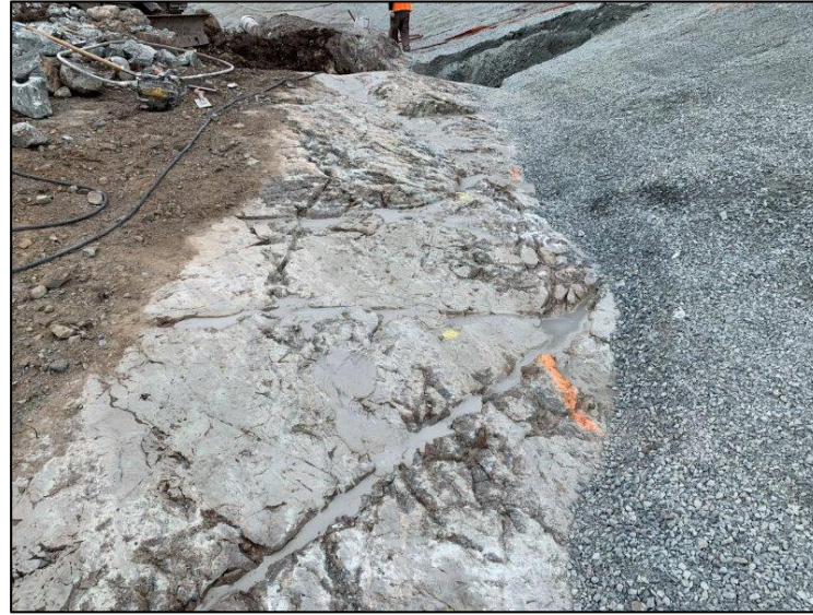
Grouting cracks. June 24, 2019
