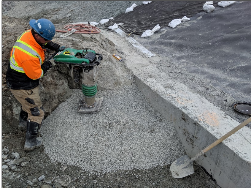
Placement of bentonite crush. July 17, 2019
