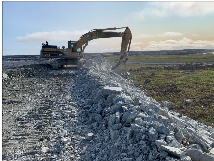
Downstream slope final shaping. July 28, 2019
