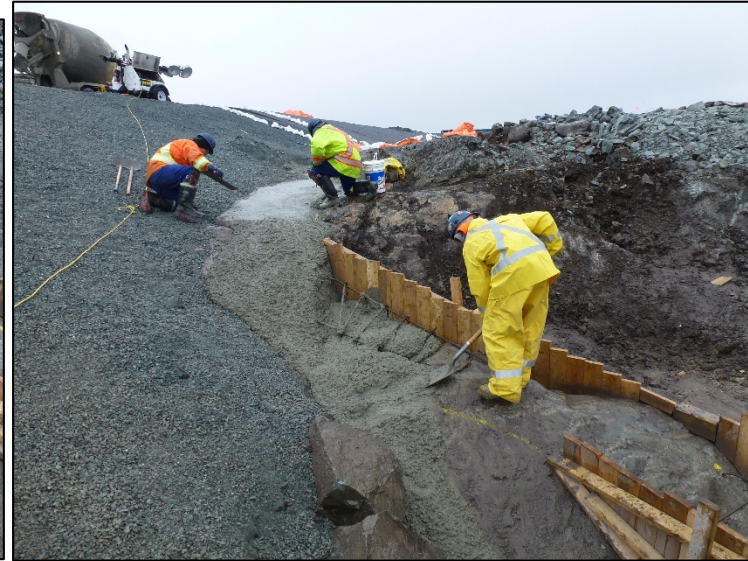
Concrete being cast from plinth to plinth 2 June 30, 2019
