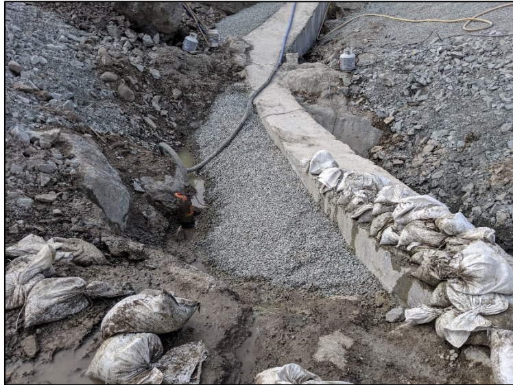
Placement bentonite crush July 17, 2019
