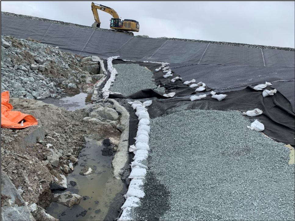
Geotextile and crush placed over liner due to ground water below liner 0+000 to 0+050. July 25, 2019
