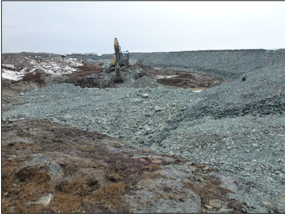
Placement of additional ROQ to fill deeper than expected overburden 0+050 to 0+075. June 14, 2019
