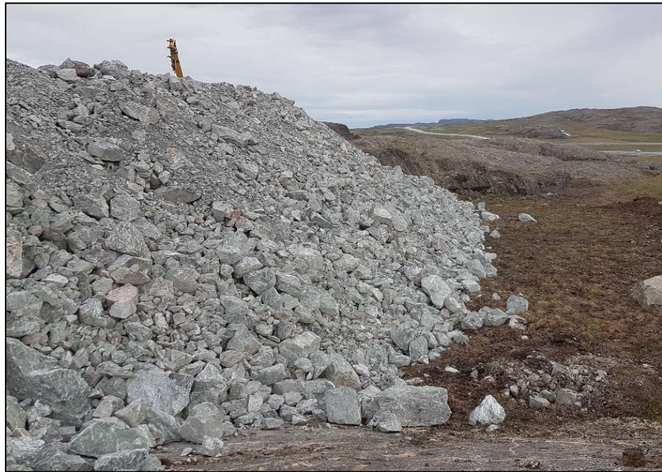
Downstream slope prior to final shaping. July 6, 2019
