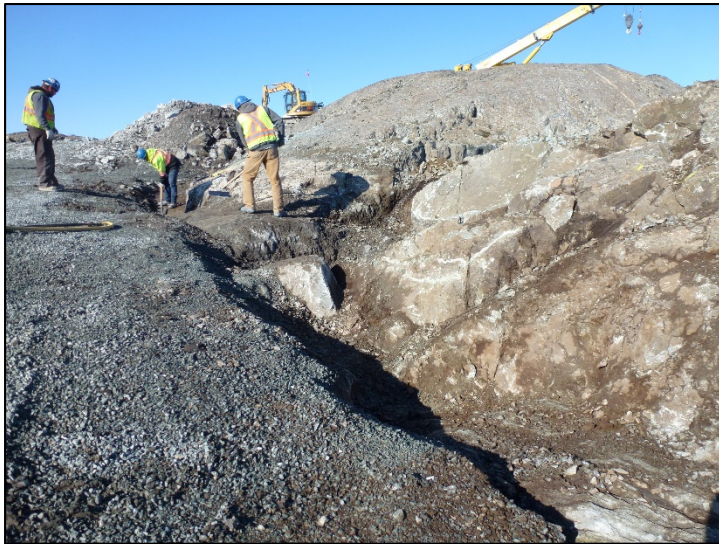
Cleaning of bedrock at liner tie-in or plinth contact 0+000 to 0+050. June 27, 2019
