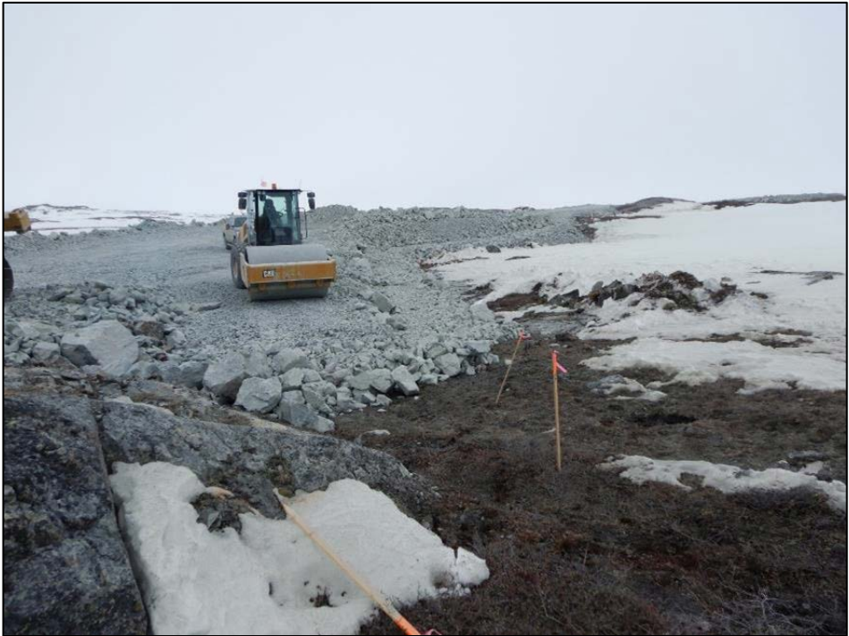
ROQ placement and roller compaction. June 3, 2019
