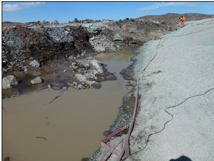
Placement of bedding material 0+160 to 0+225. June 25, 2019
