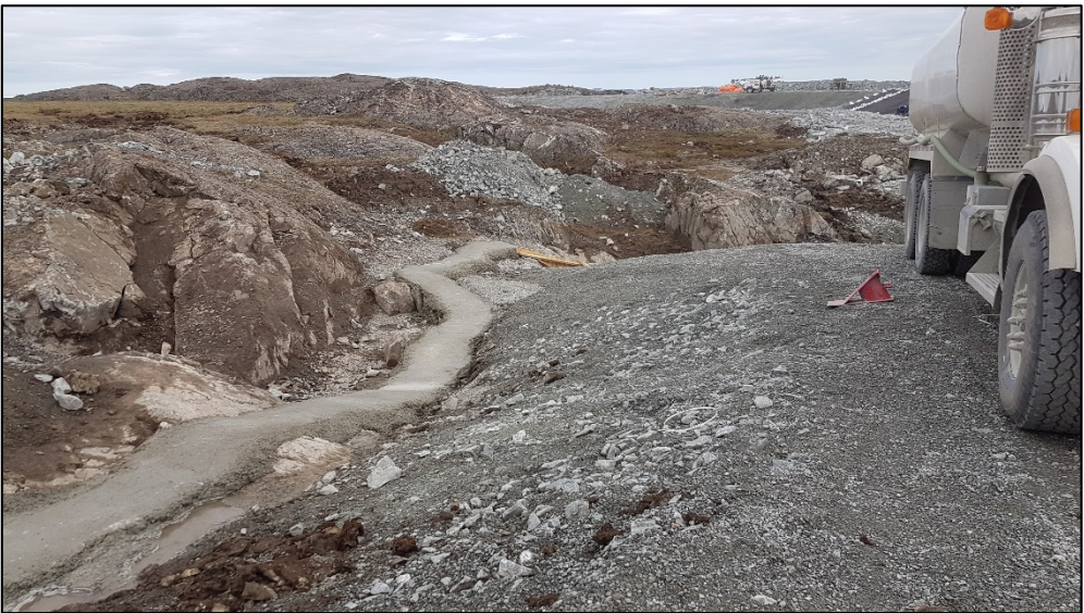
Concrete grouting for liner tie-in 0+000 to 0+50. July 3, 2019
