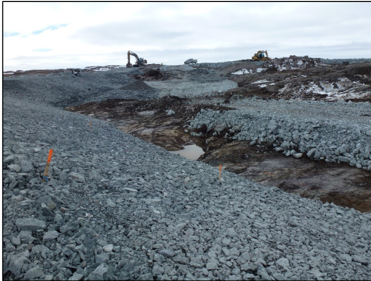
Placement of transition material 0+000 to 0+100. June 16, 2019
