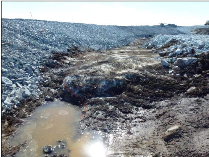
Excavation of overburden at upstream toe to expose Bedrock 0+100 to 0+0+160. June 13, 2019
