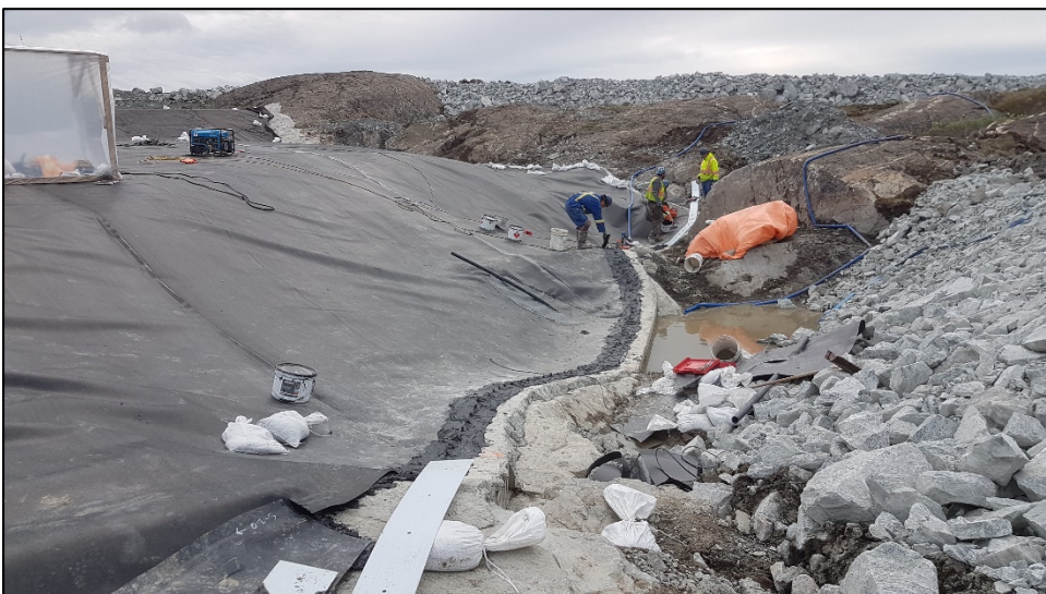
Liner placement and tie-in 0+000 to 0+100. July 8, 2019
