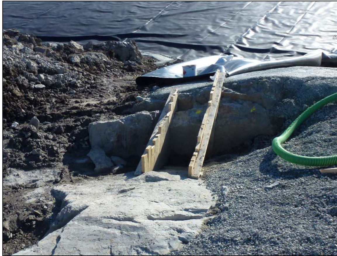
Contact rock cleaned and formwork placed plinth 9. July 2, 2019
