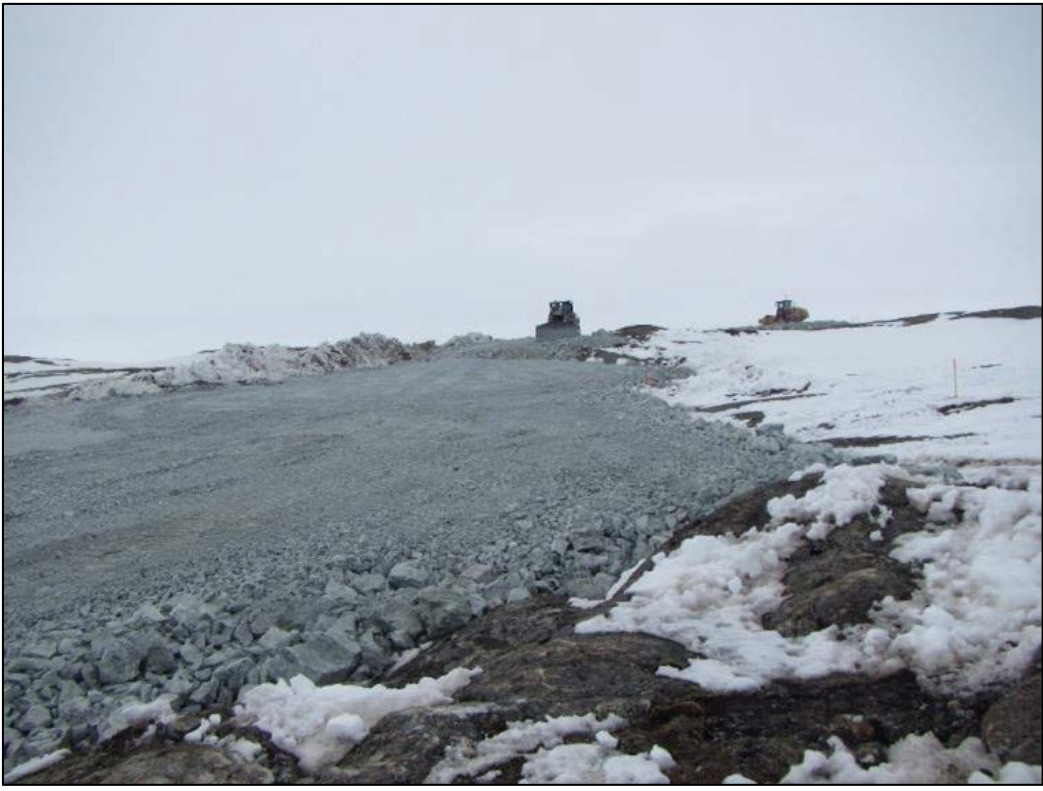
ROQ placement. May 30, 2019 Note: Photo provided by TMAC site personnel.
