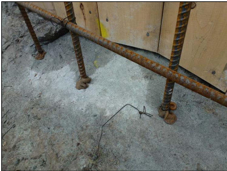
Steel reinforcing secured in bedrock. June 30, 2019
