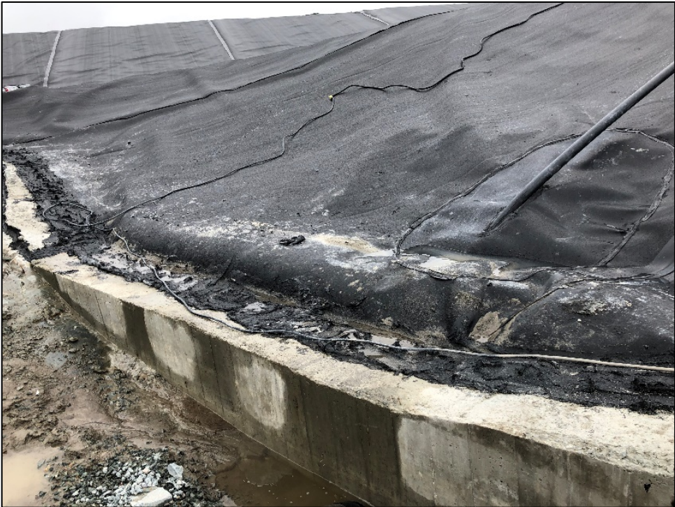
Liner pushed up by water 0+000 to 0+050 July 11, 2019
