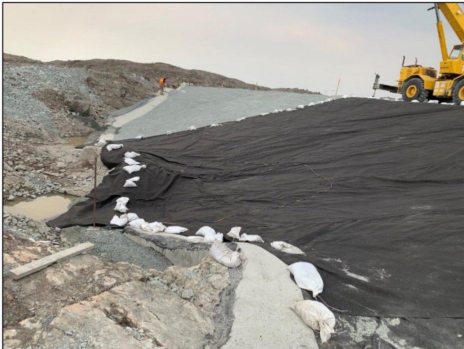
Geotextile placement 0+160 to 0+225. July 25, 2019
