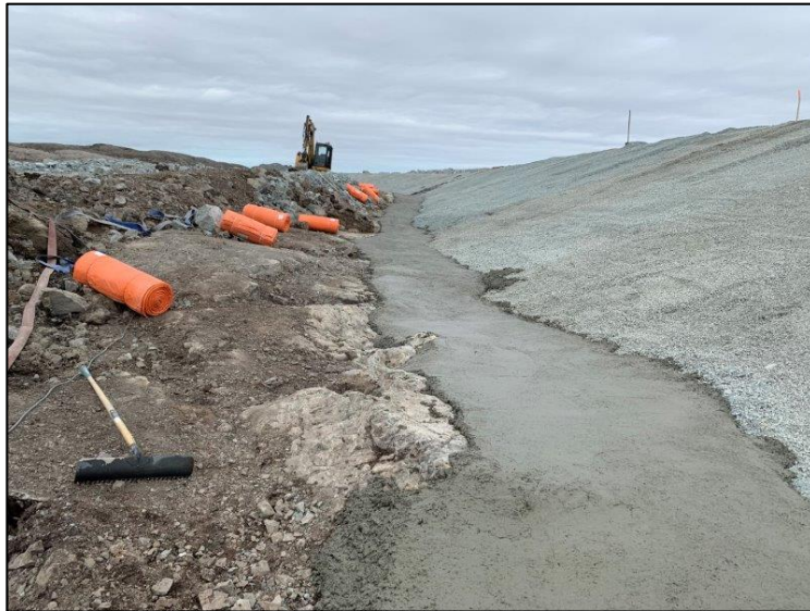
Concrete liner tie-in 0+100 to 0+160. June 24, 2019
