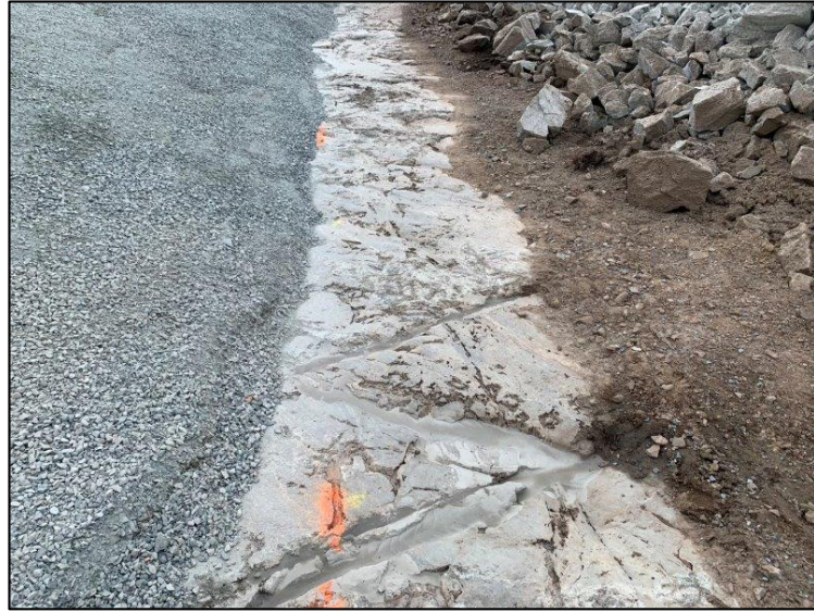
Grouting cracks. June 24, 2019
