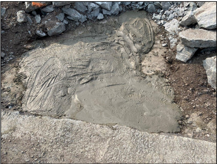
Crack/void grouted. July 25, 2019
