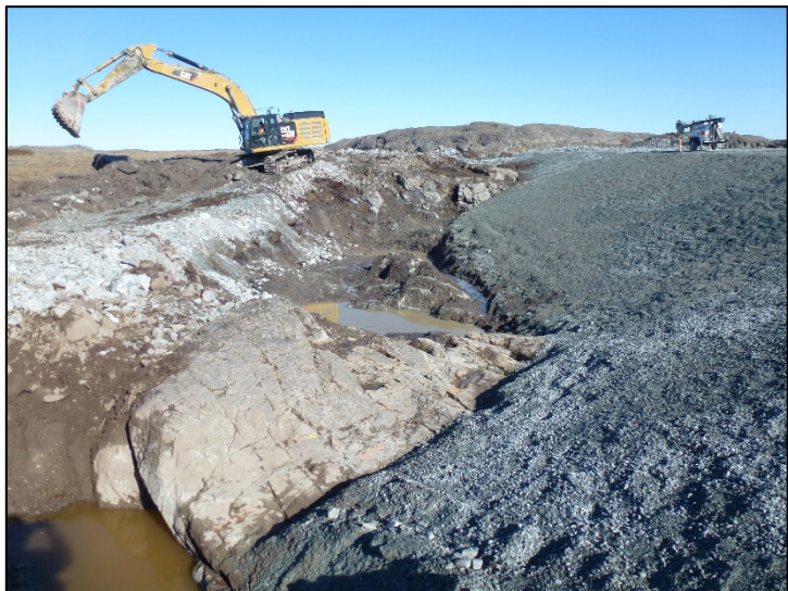
Cleaning of bedrock at liner tie-in or plinth contact 0+160 to 0+225. June 27, 2019
