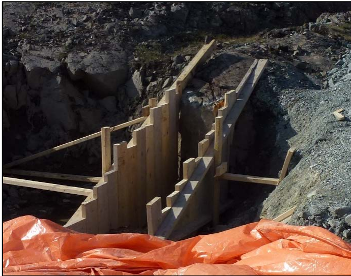
Formwork for plinth 8. June 29, 2019
