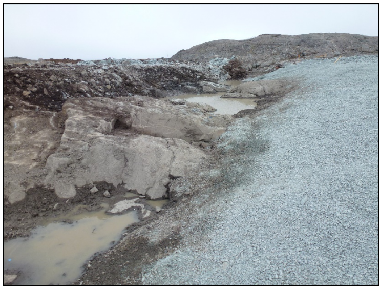
Cleaning of bedrock at liner tie-in or plinth contact 0+160 to 0+225. June 26, 2019
