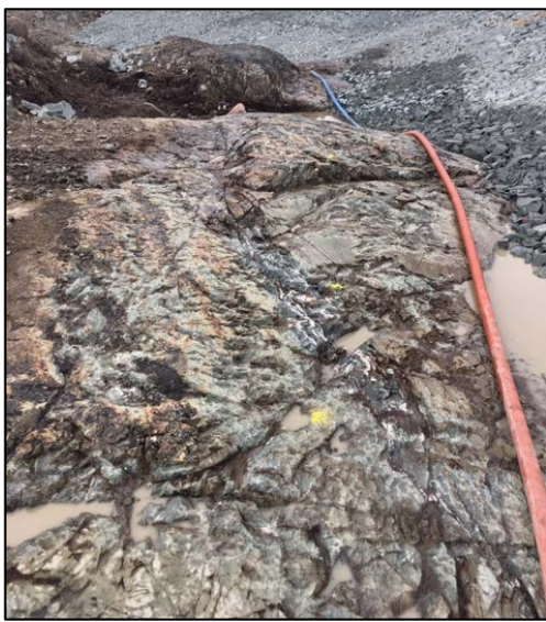
Cleaning of bedrock at liner tie-in or plinth contact 0+100 to 0+160. June 20, 2019
