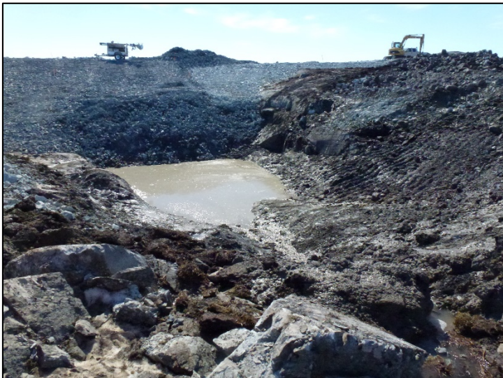
Excavation of overburden at upstream toe to expose Bedrock 0+000 to 0+100. June 13, 2019
