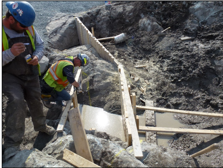
Formwork for plinth 2 & 3 contact. June 29, 2019
