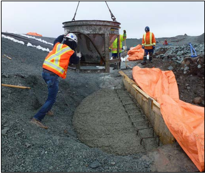
Concrete being cast for plinth 1 June 30, 2019
