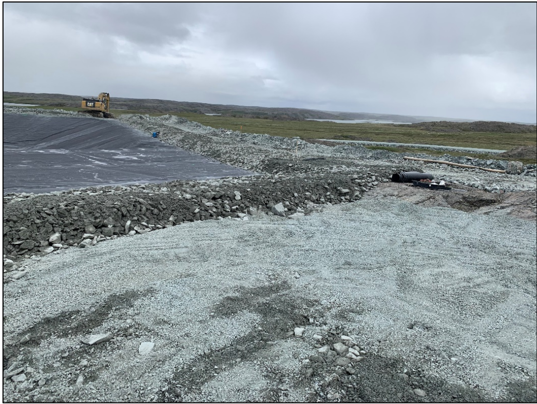
Liner anchor material 0+050 to 0+160. July 28, 2019
