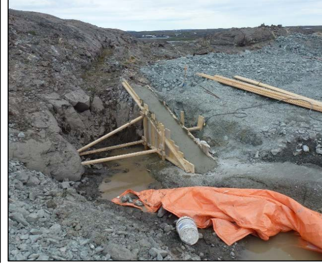
Concrete cast plinth 8 July 2, 2019
