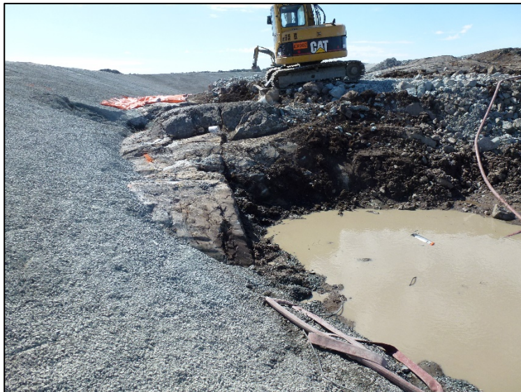
Placement of bedding material 0+100 to 0+160. June 25, 2019
