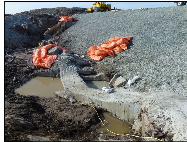
Formwork stripped plinth 2 and plinth 3 July 1, 2019
