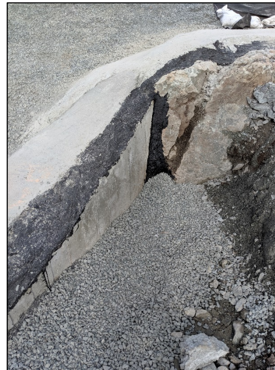
Sopramastic and bentonite crush placed July 17, 2019
