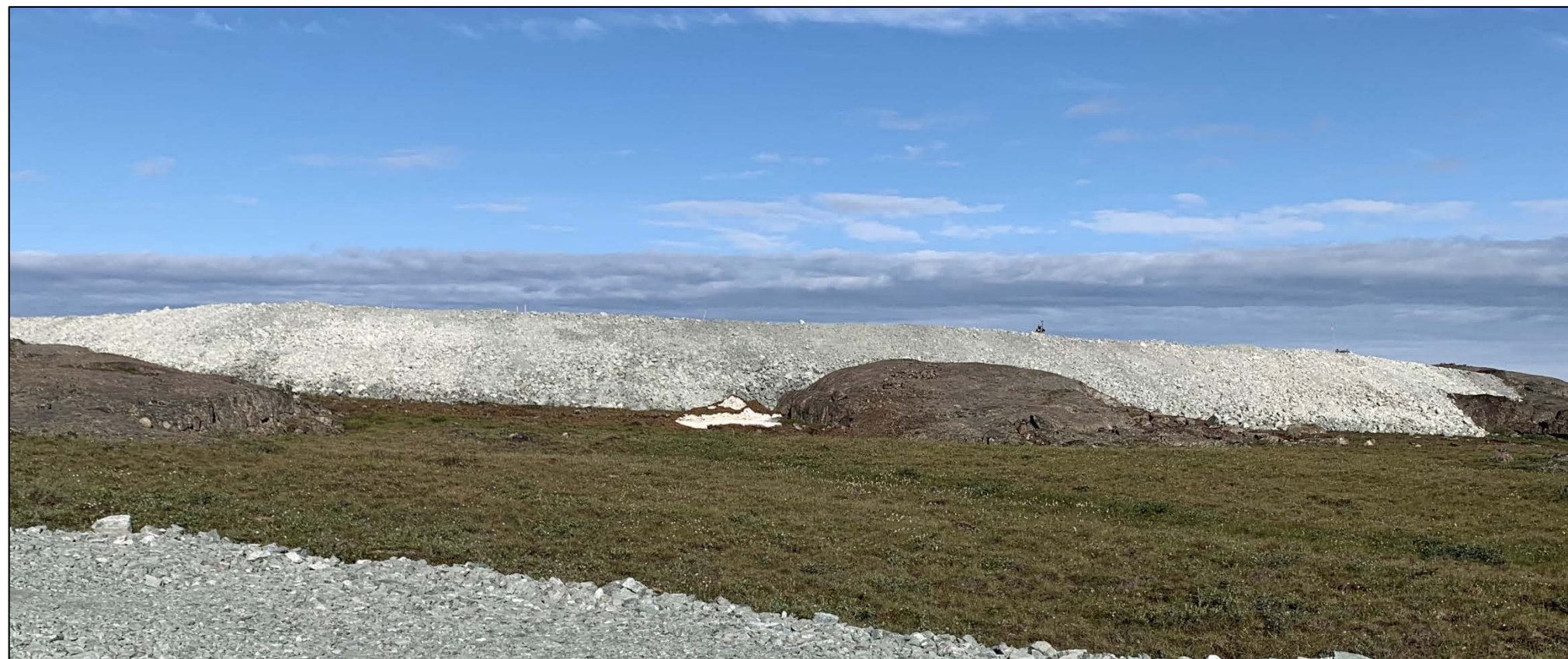
Downstream slope final shaping. July 28, 2019
