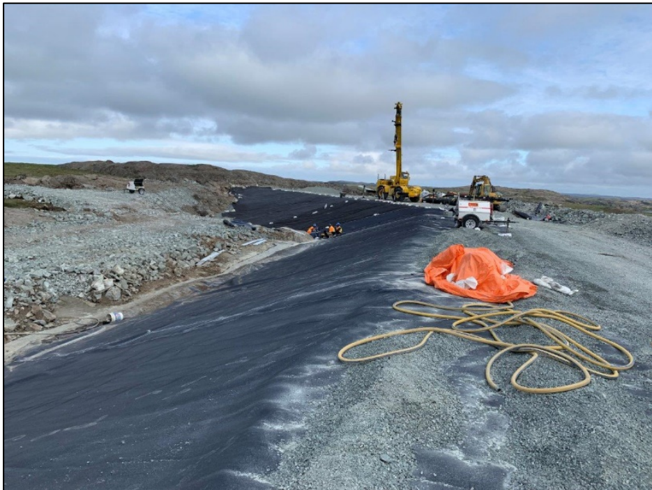
Geotextile and liner placement 0+160 to 0+225. July 25, 2019
