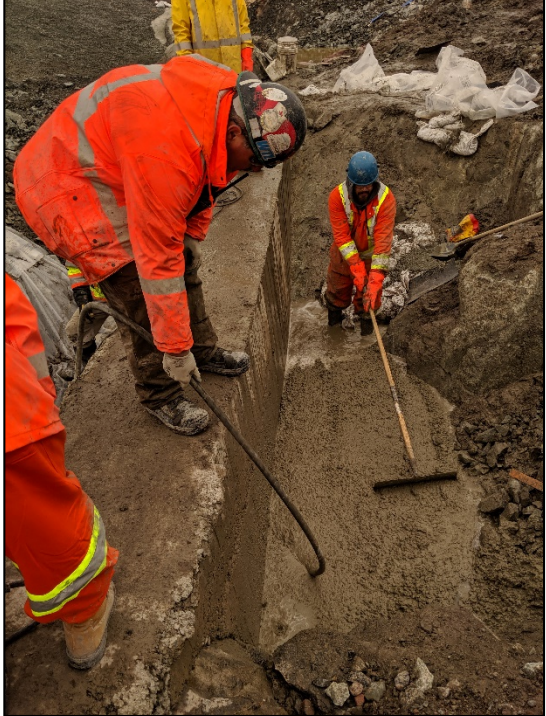
Concrete grouting cast. July 13, 2019
