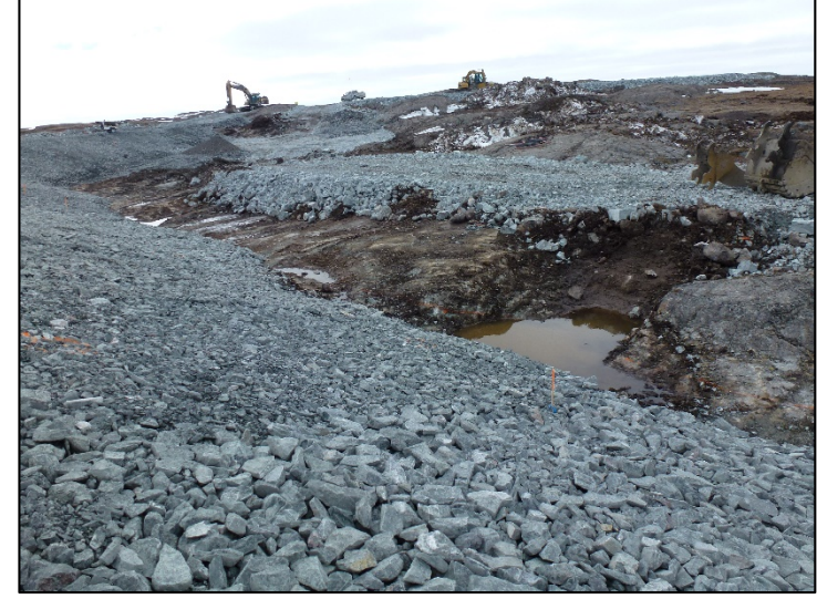
Excavation of overburden at upstream toe to expose Bedrock 0+100 to 0+160. June 17, 2019
