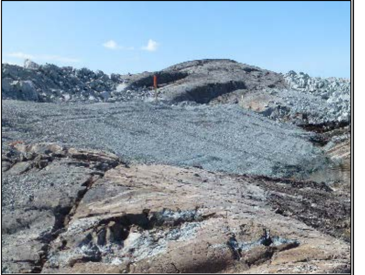
Placement of bedding material 0+000 to 0+050. June 25, 2019
