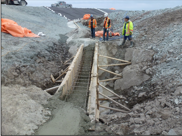
Concrete casting plinth 4. July 2, 2019
