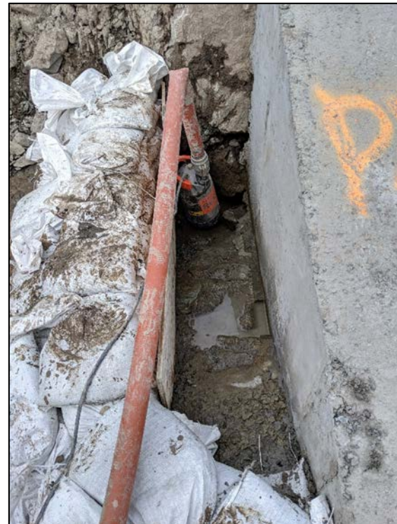
Voids cleaned and formwork for concrete grouting. July 15, 2019
