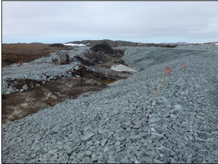
Placement of transition material 0+100 to 0+160. June 16, 2019
