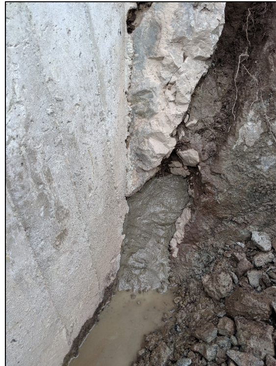
Placement of Sikaset Plug within void. July 16, 2019
