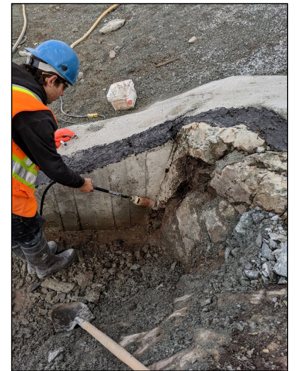
Drying surfaces prior to applying patch material. July 16, 2019
