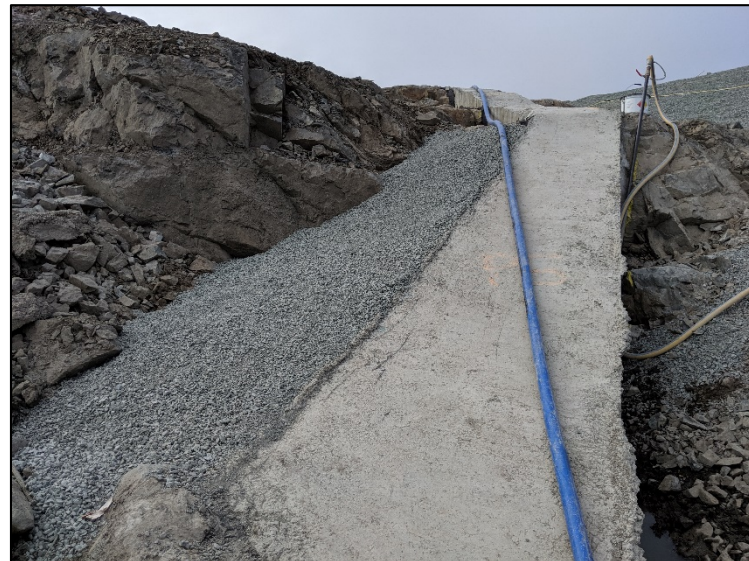
Bentonite crush placed. July 17, 2019
