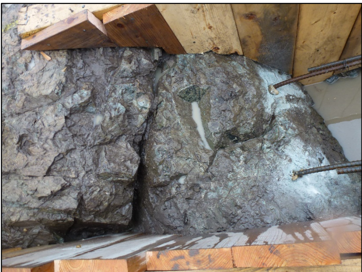
Steel reinforcing secured in bedrock plinth 7. June 30, 2019
