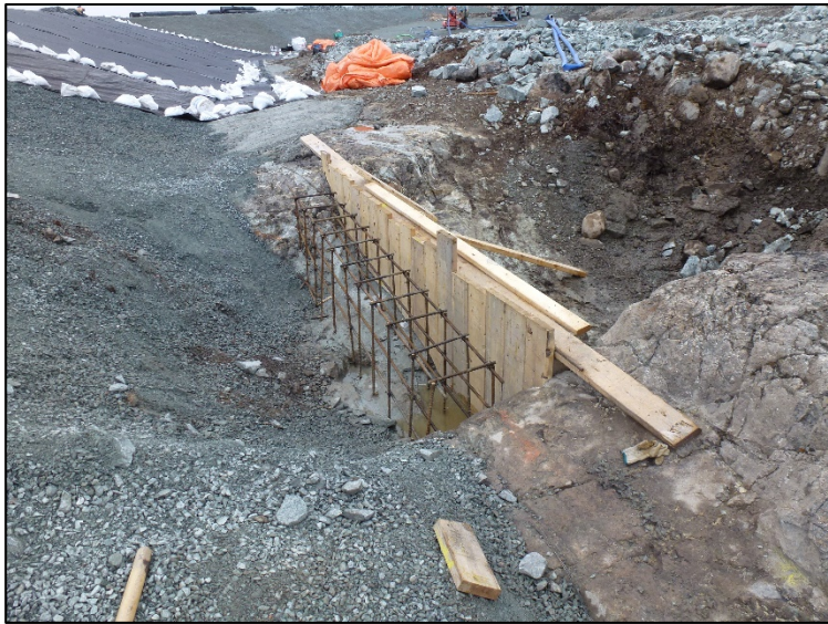
Formwork and steel reinforcing for plinth 1. June 30, 2019
