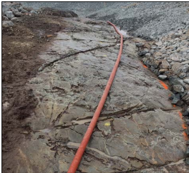
Cleaning of bedrock at liner tie-in or plinth contact 0+100 to 0+160. June 20, 2019
