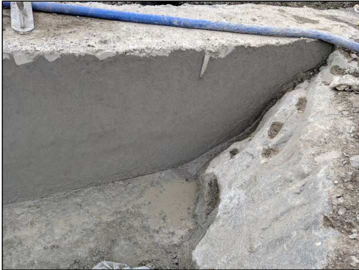
Seal al joints with Sika Sikaset Plug plinth 4. July 14, 2019
