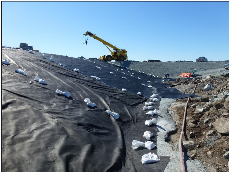
Geotextile and liner placement 0+050 to 0+100. June 28, 2019
