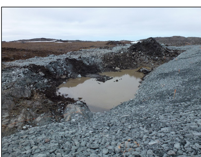
Excavation of overburden at upstream toe to expose Bedrock 0+160 to 0+225. June 17, 2019
