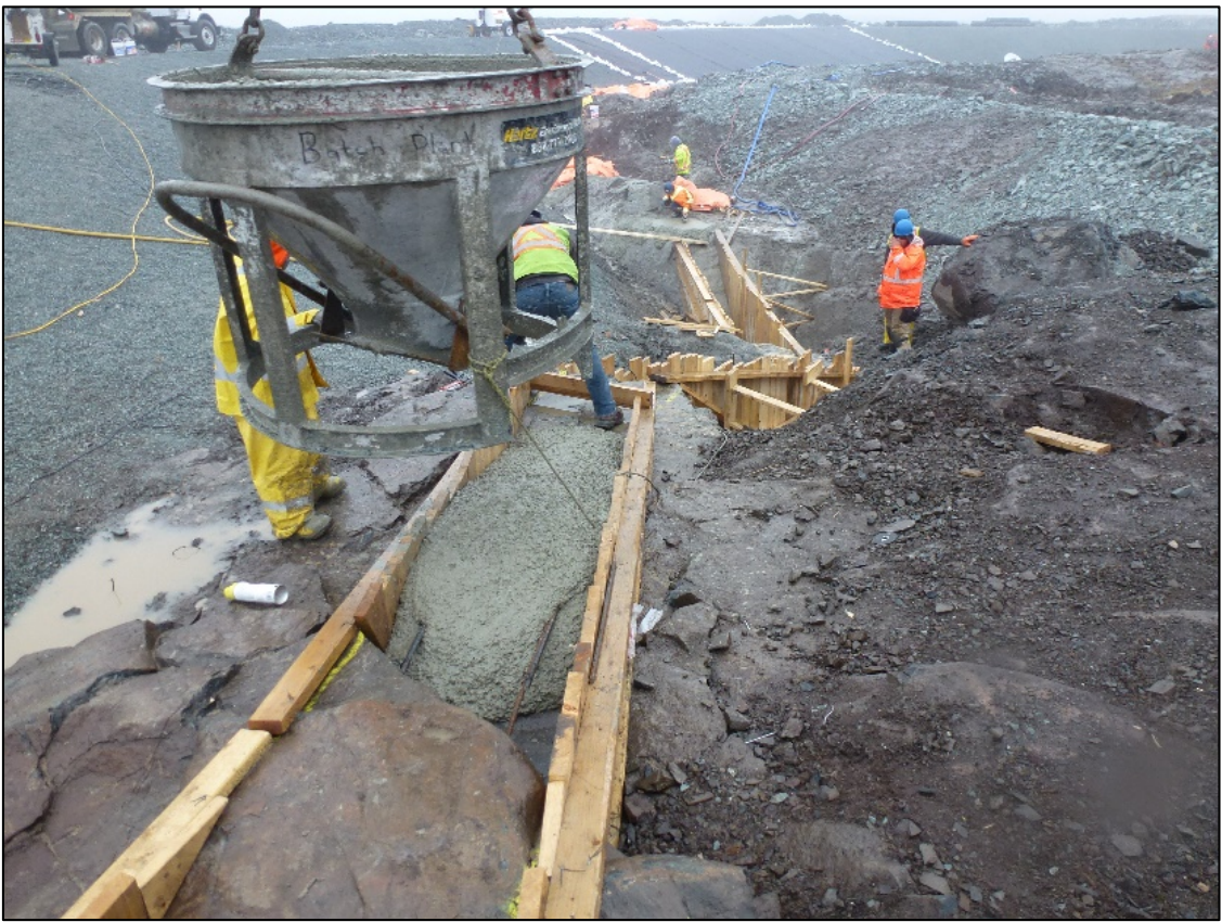
Concrete casting plinth 6 June 30, 2019
