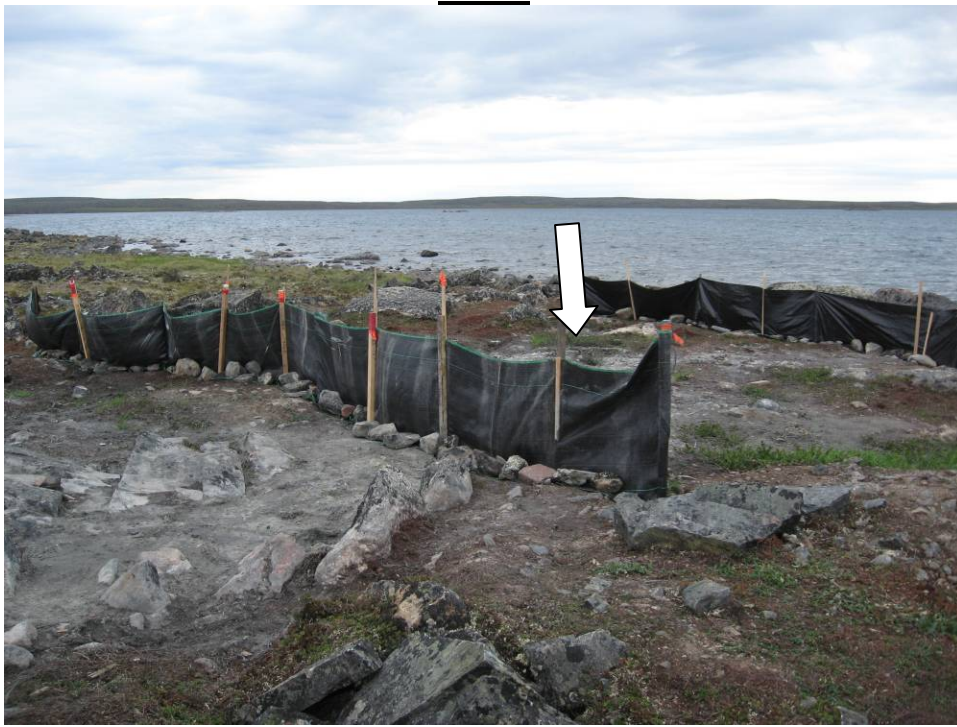
Removal by shovelling of drill cuttings between the two silt fences
