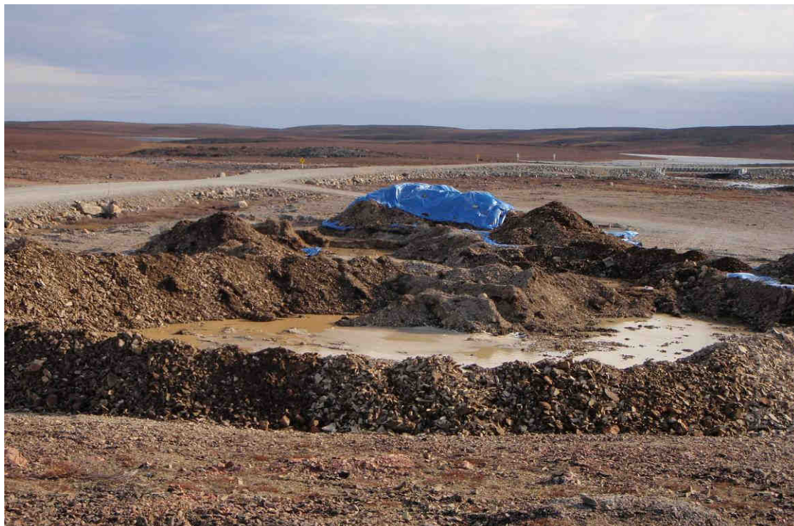
Photo 01: After completion of the contaminated soil exhumation last falls, banks on each side of the holes have been created to avoid any incident. – September 23 rd 2008
