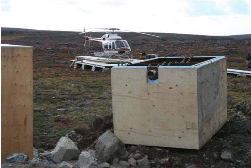
3. Grease trap before the installation ; isolated 4' x 4' x 6'.
