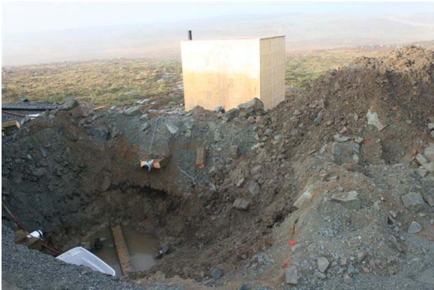
1. Construction of the new grease trap.
