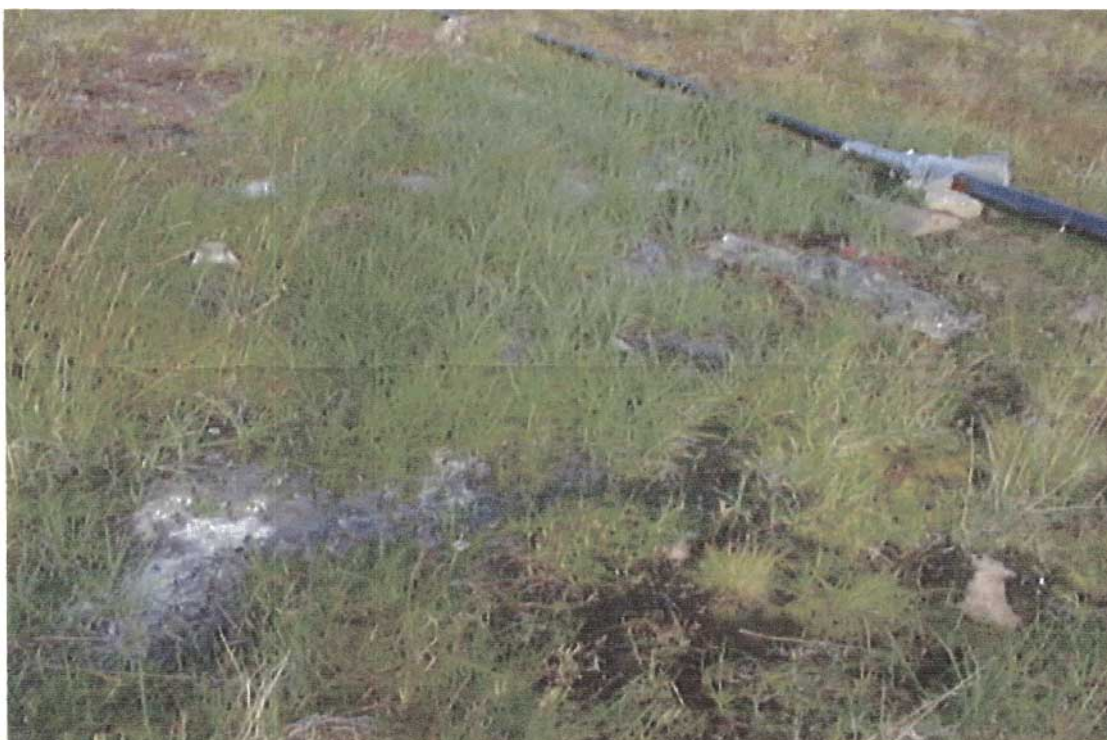
figure 3. Break in greywater discharge line; 2000/08/30.
