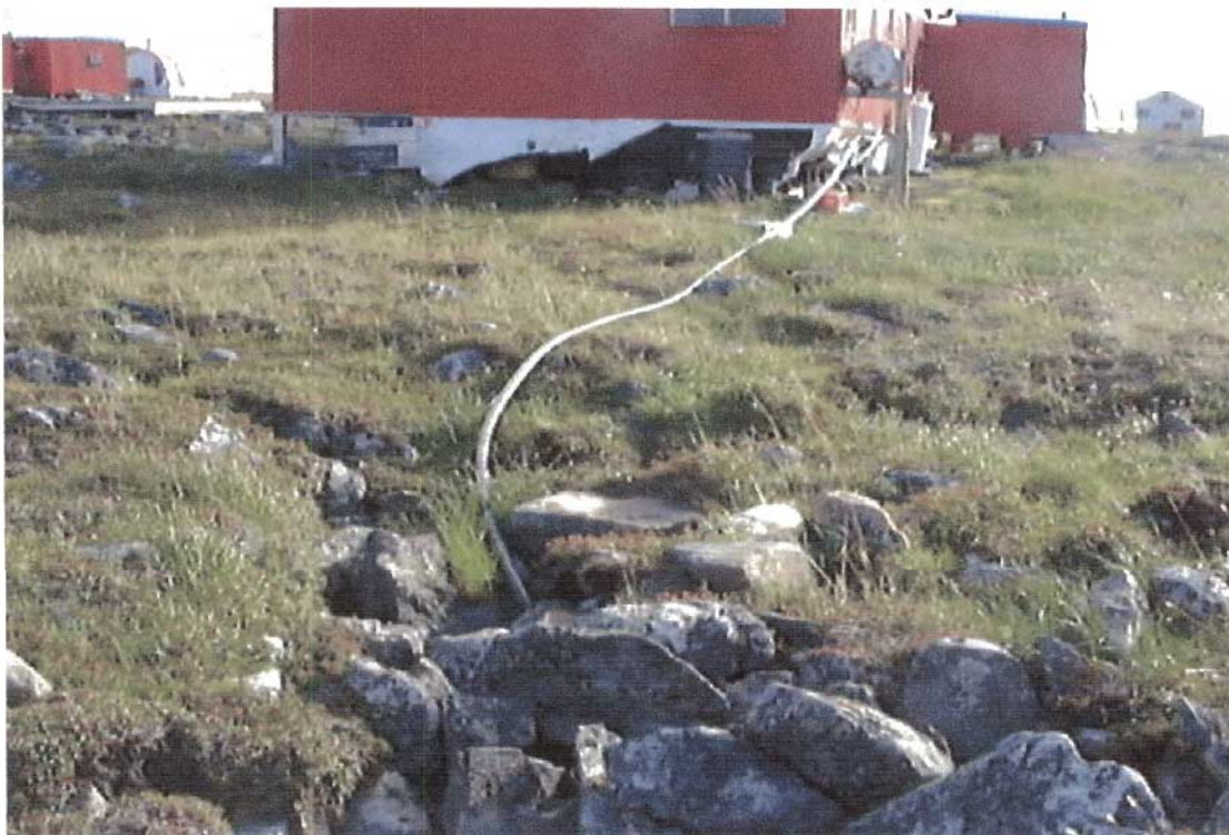
figure 2. Greywater sump; 2000/08/30.
