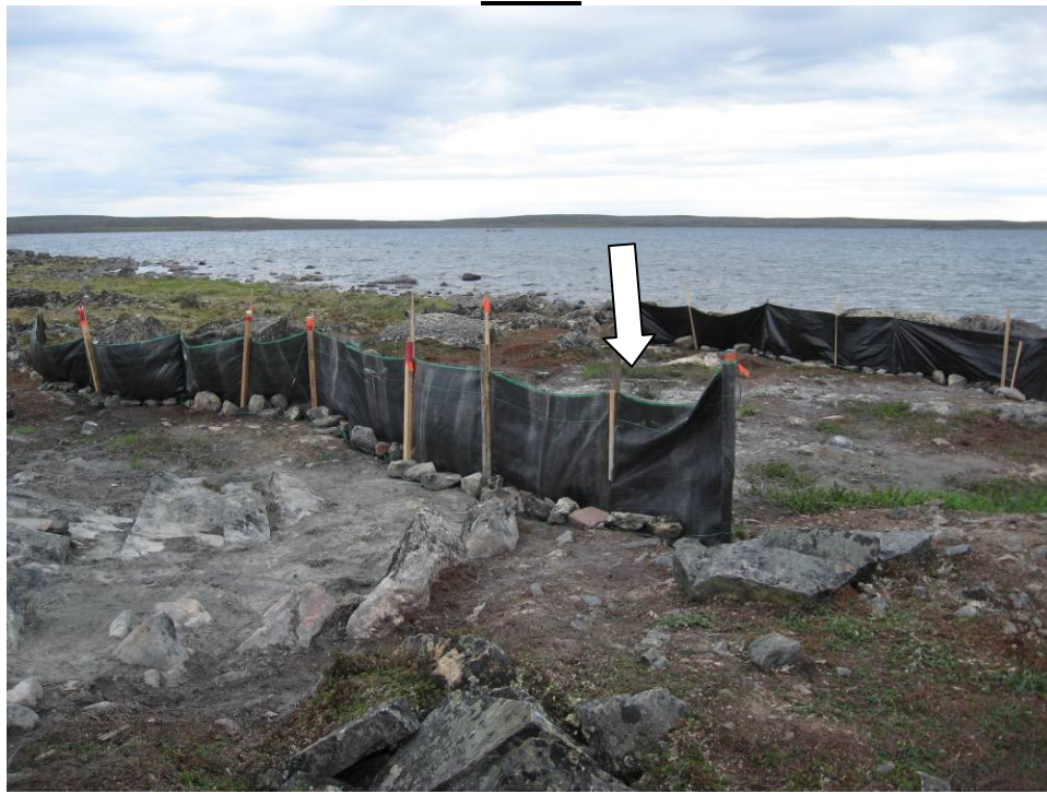
Removal by shovelling of drill cuttings between the two silt fences
