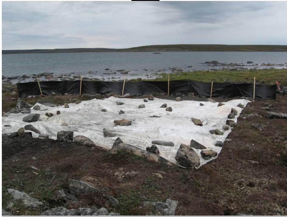
Silt fence and waterproof membrane to prevent rain erosion
