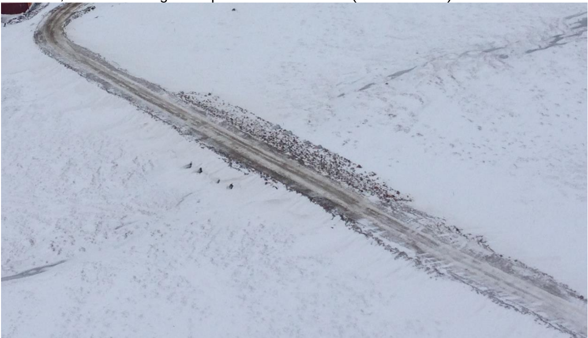
Picture 4, Water crossing with upstream stabilization (October 2015)
