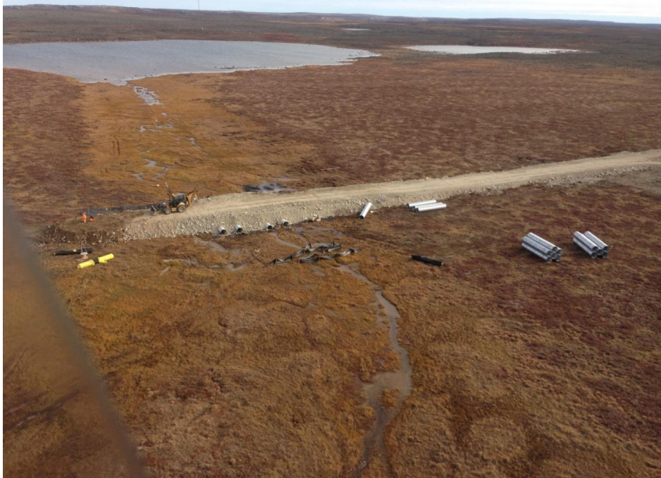
Picture 1, Crossing 181 during construction (September 2015)
