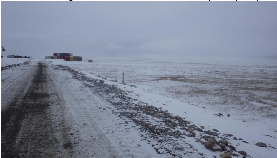
Picture 3, Crossing 181, downstream stabilization completed (2016)
