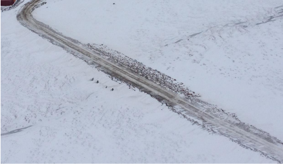
Picture 2, Crossing 181, upstream stabilization completed before winter (October 2015)
