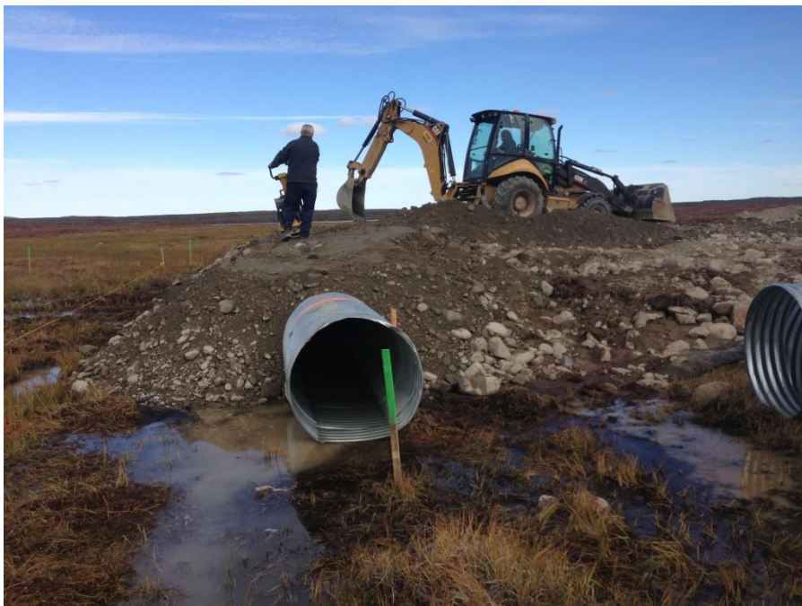
PHOTO 4 Backfilling and compacting
