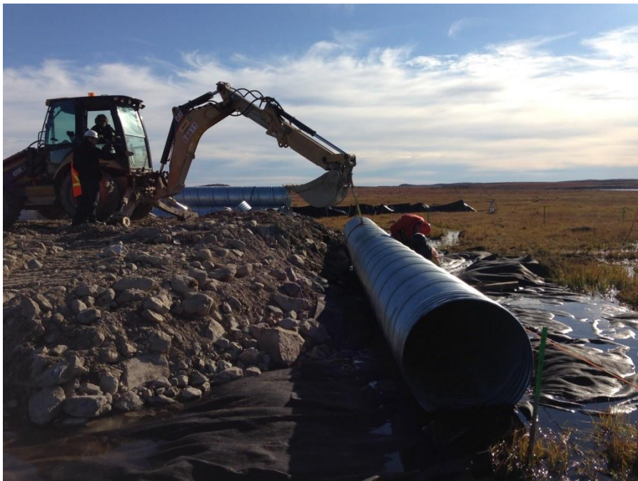
PHOTO 2 Installation of the first culvert
