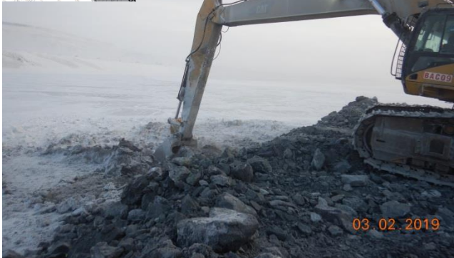
Photo 3: Removal of ice with an excavator
