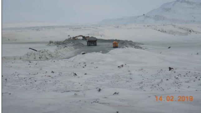
Photo 6: permeable berm construction. Excavator is broken the ice before the dozer advance the structure
