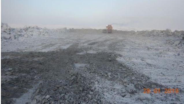
Photo 5: Permeable berm rockfill placement
