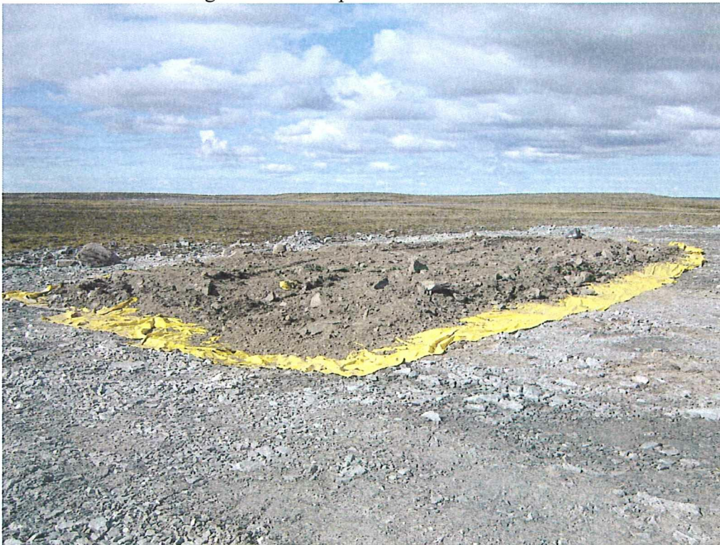
Plate 1B: Land farming of soils on Operations Pad
