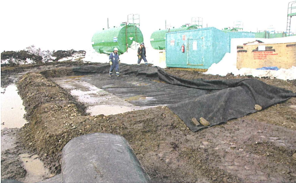
Plate 1B: Land farming of soils on Operations Pad
