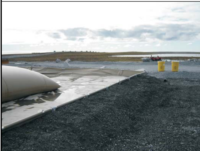
1E: Operations Pad: Completed bladder/instaberm installation with lined fueling station in middle ground
