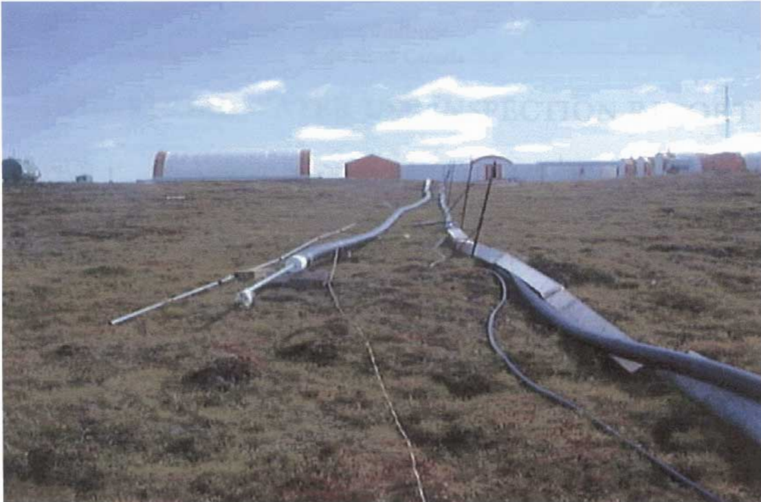
figure 1. Replacement of the water supply conveyance line; 2001/08/28.
