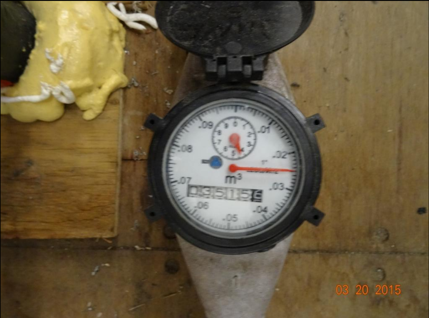
Description: Top picture # 1565: Indirect water use meter, location in the fresh water treatment room. Bottom picture # 1566: Flow meter reading.
