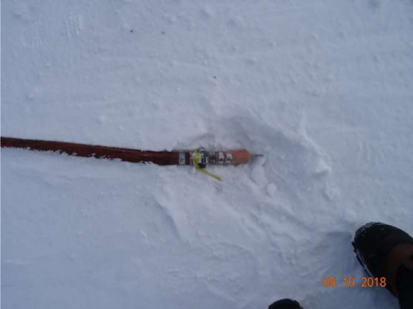
Description Water supply hose frozen into the ice. A rope has been tied to in so that it can be removed in the summer.
