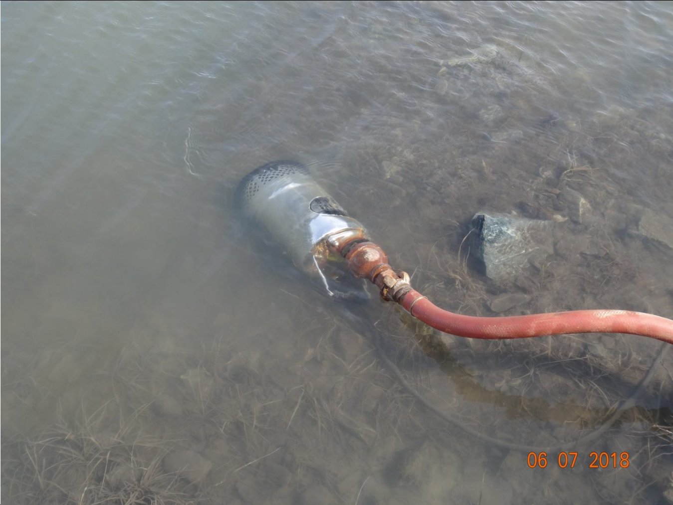
Description: Drill 1: Reclaim water source, screened water intake.
