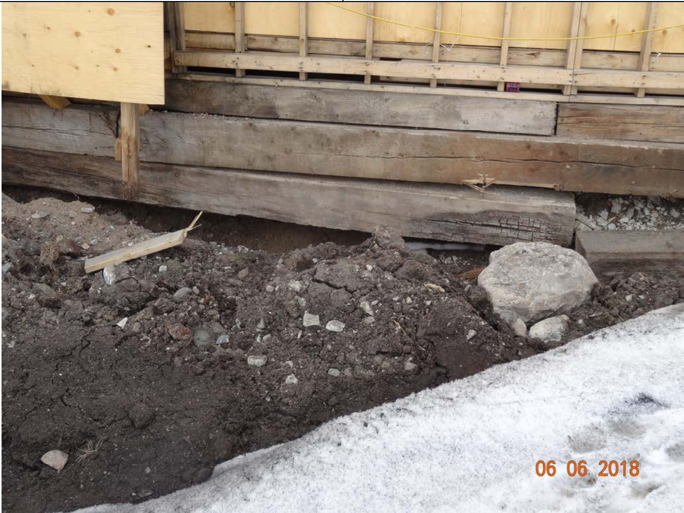
Description: Stained ground under genset building.
