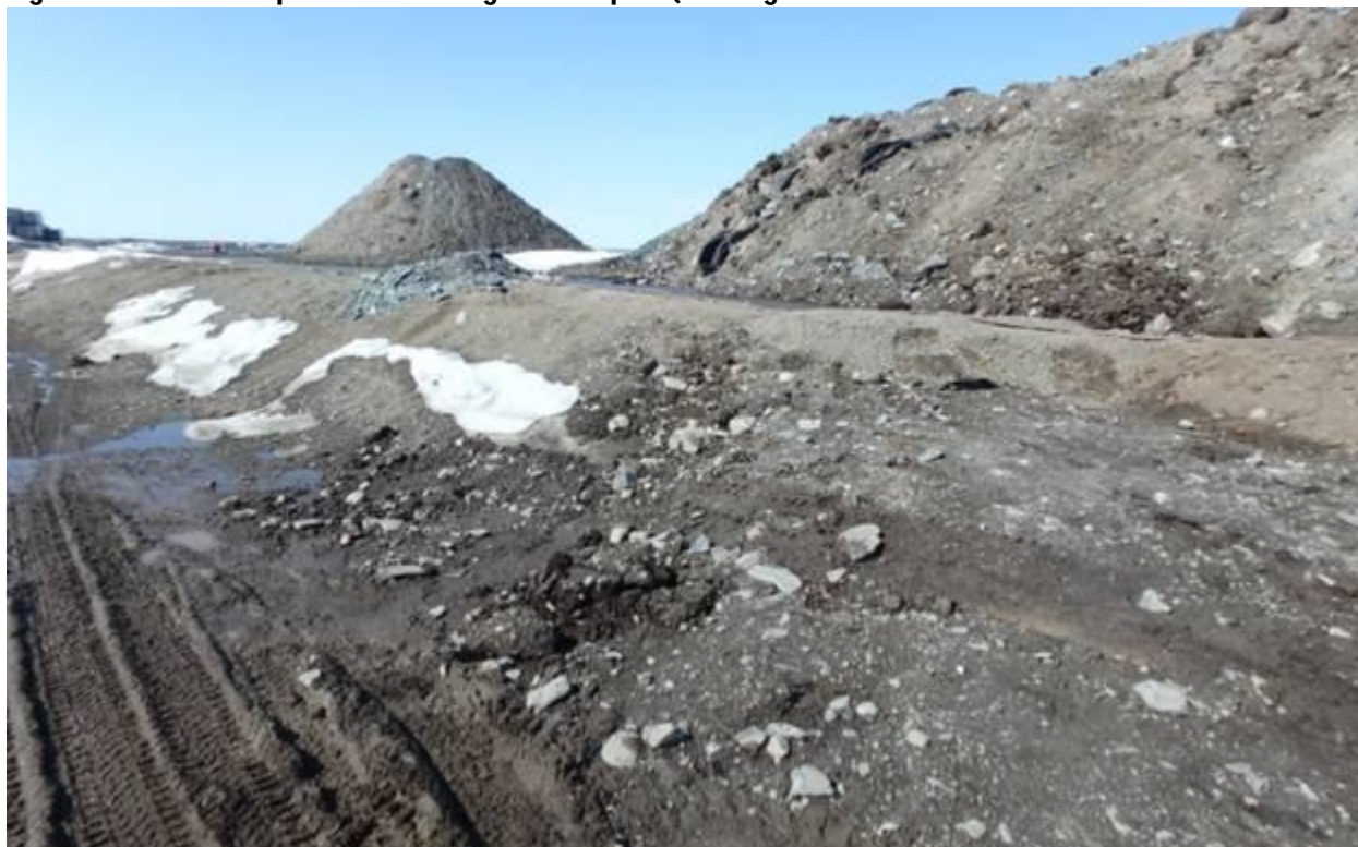
Figure 3: Raised ramp and containing berm repair (looking northeast from west side of landfarm berm)
