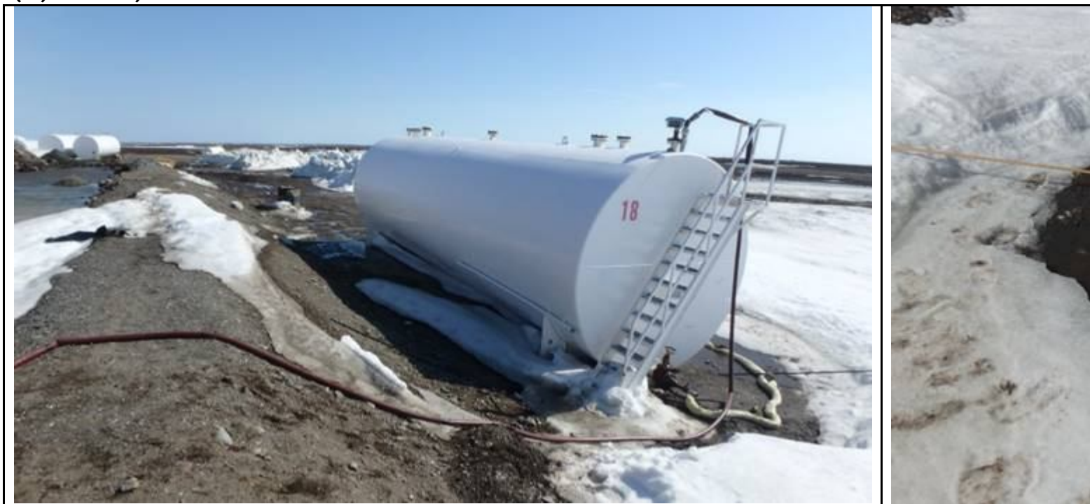
Figure 2a and 2 b: Absorbent boons placed downstream of snow melt under fuel storage tank (looking (2a) south and (2b) northeast)
