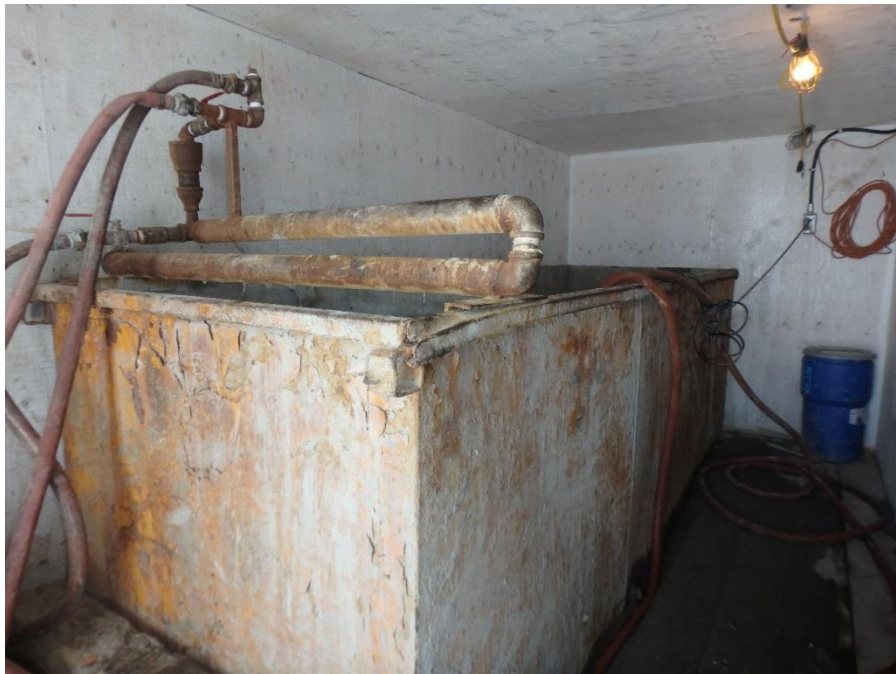
Figure 2, Waste water settling tank
