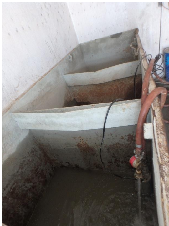
Figure 3, Waste water settling tank
