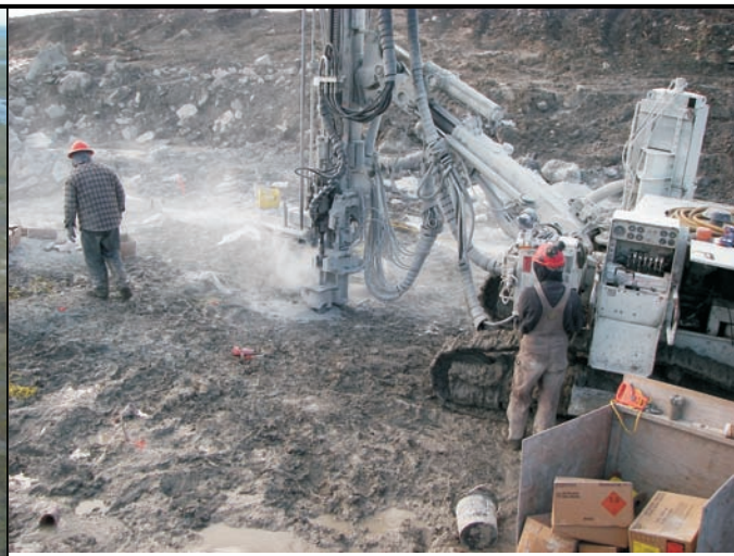
2B: Airtrack Drilling - Portal Boxcut - October 2007
