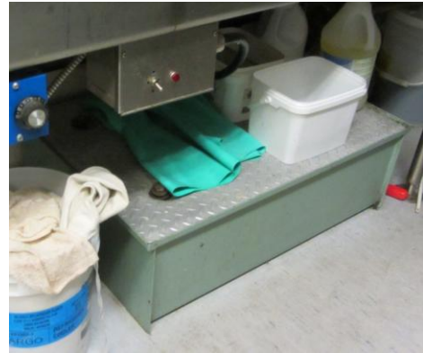
Photo 1. In-line grease interceptor
