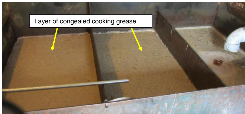
Photo 2. Large grease trap in kitchen discharge line.
