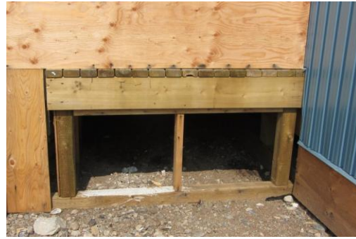
Photo 33. Section of skirting removed and not replaced.
