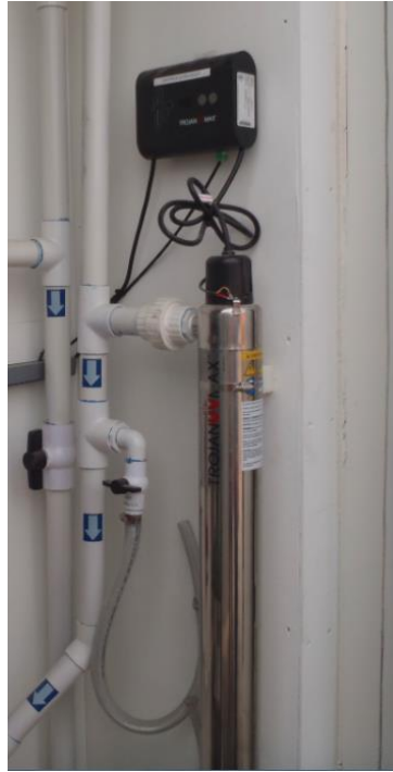
Illustration 8 : Disinfection unit
