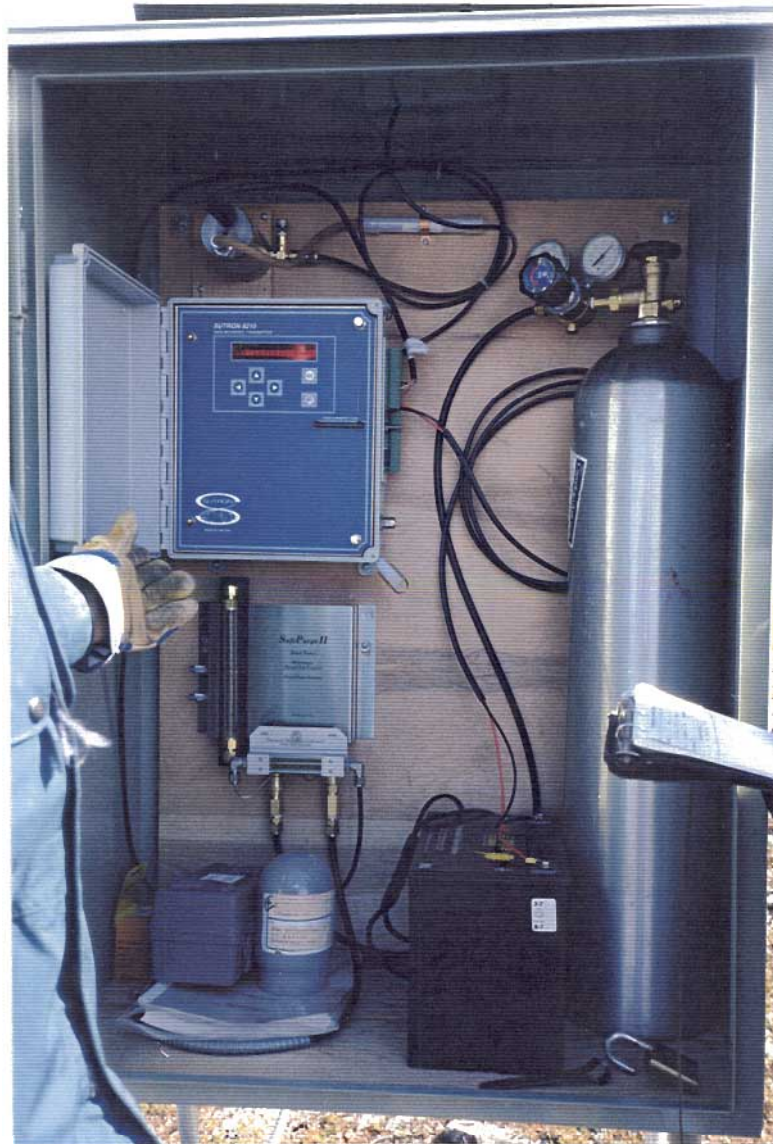
Photo 33. Automatic water level monitoring station, equipment inside shelter.
