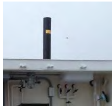
Figure 2: installation of the vent
