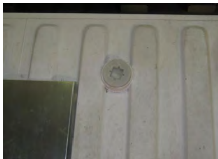
Figure 2: installation of the vent
