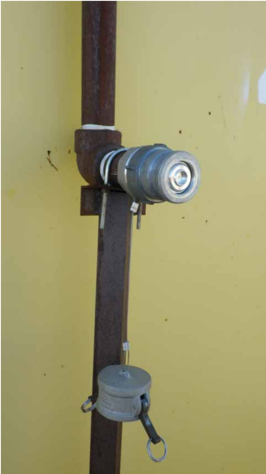
Jet A Tank CAMLOCK FITTING at Meliadine Location
