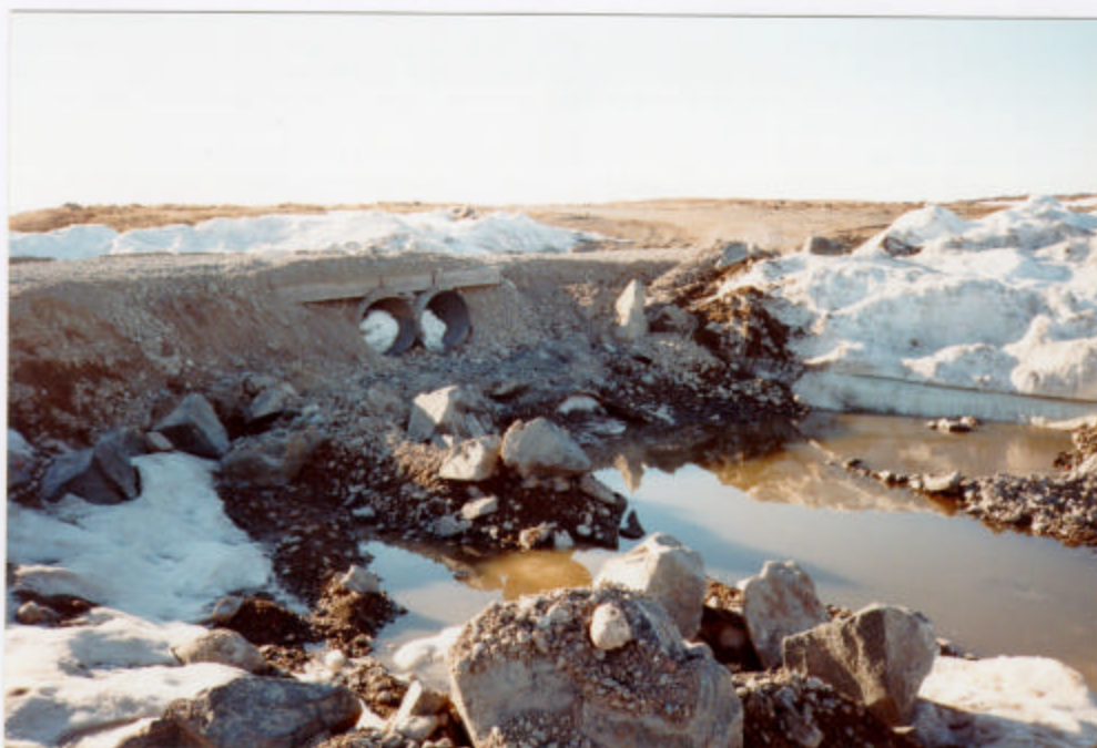
Photo 2: June 12, 2000. Char River road crossing; ponded water at downstream end. The lower culvert is completely blocked with snow and ice; the two upper culverts are at least partly blocked.
