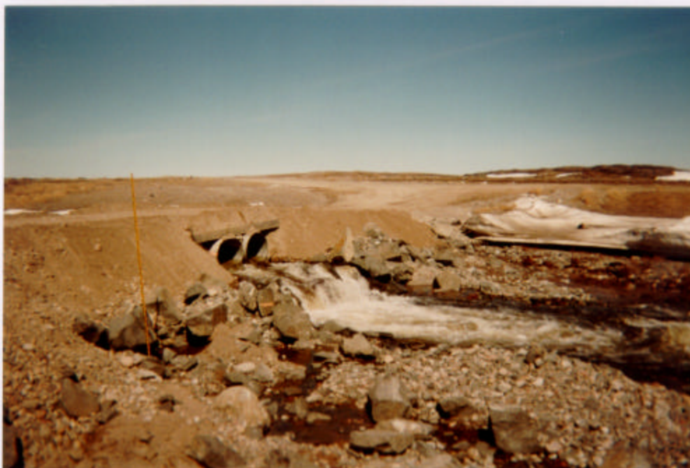
Photo 7: June 21, 2000. Char River at road crossing; looking at culvert outlet. Road was re-instated on June 20. Discharge is 4.4 \text{ m}^3/\text{s} , through the two upper culverts only; the lower culvert is still blocked.
