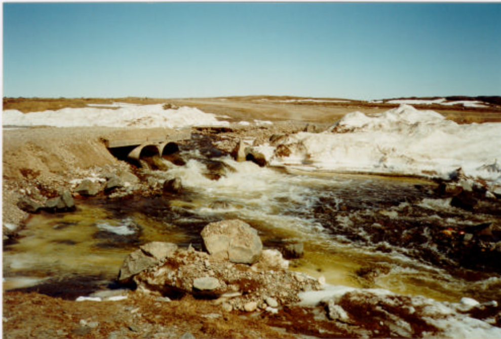
Photo 6: June 14, 2000. Char River road crossing looking upstream. Discharge is 5.0 \text{ m}^3/\text{s} . Flow passing through the two upper culverts and over the left embankment.
