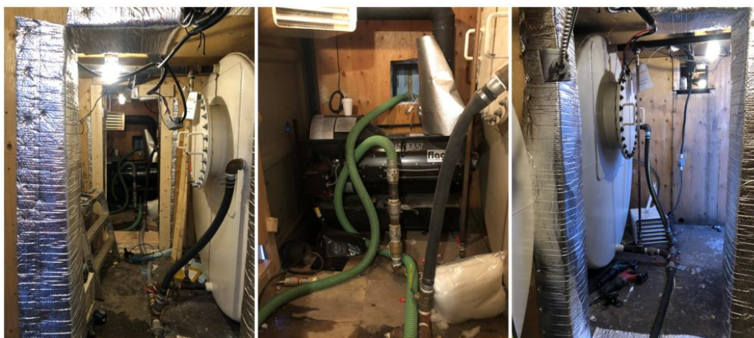
Figure 4: Improvements made to the interior of the retention tank storage containers. Four containers have been connected so that all lines running between tanks, are no longer exposed to external temperature. An additional heater was installed at ground level.
