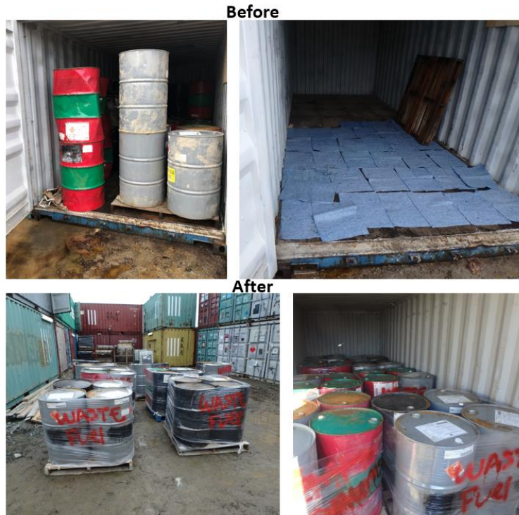
Figure 4: Condition of the seacan before, and after decontaminating and repacking the drums.
