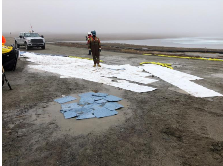
Figure 2: Initial Jet A spill initial containment.
