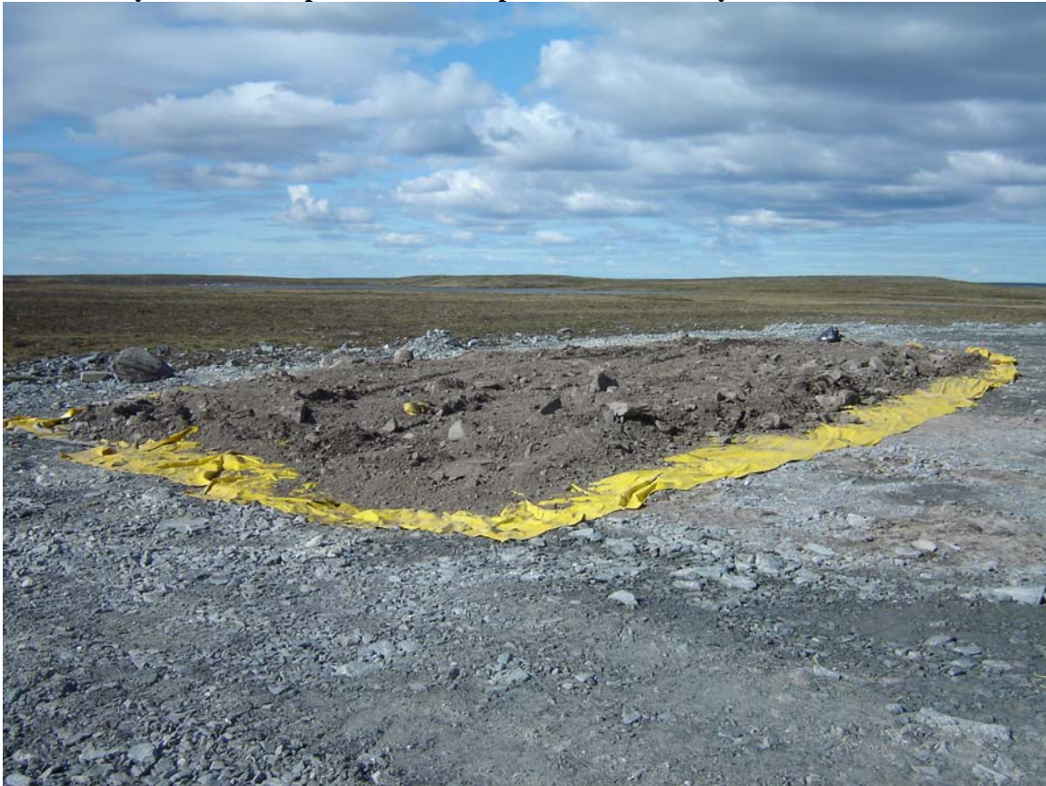
Plate 1B: Hydrocarbon impacted soils on Operations Pad – July 2008
