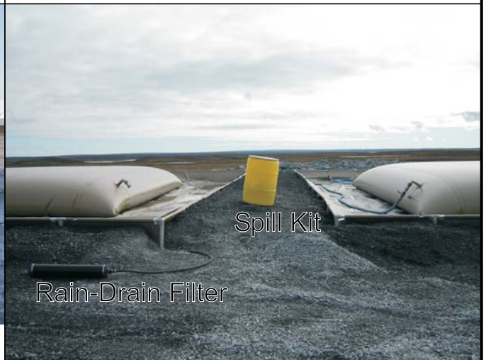
1D: Operations Pad: Completed bladder/instaberm installation with waste rock support berm
