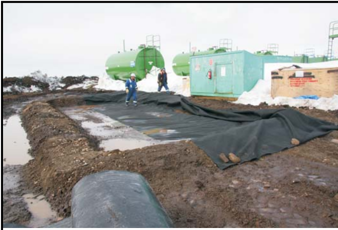
1A: Liner installation - Main Bulk Fuel Facility Fueling station
