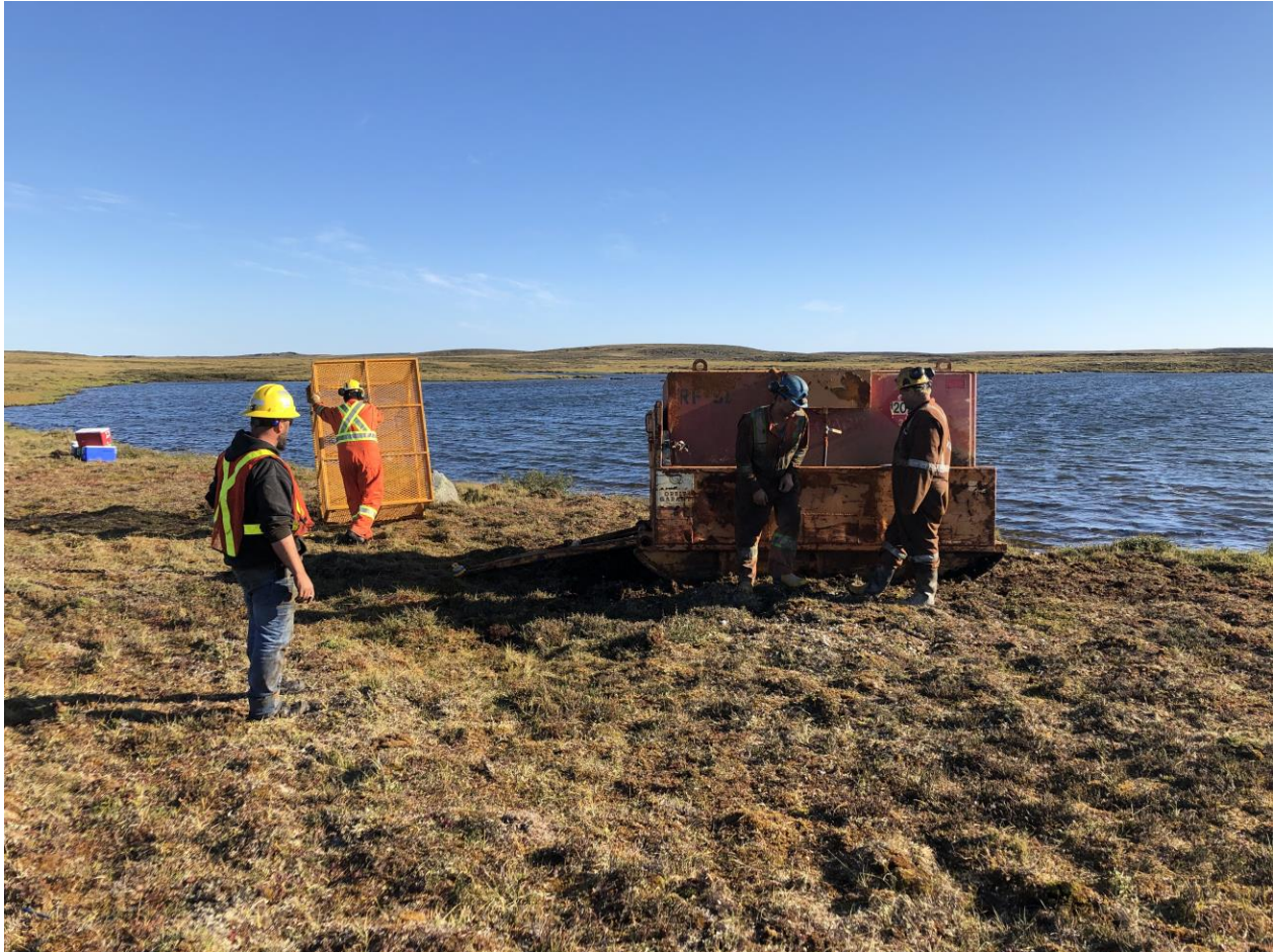
Figure 1. The fuel tank is being extracted from the lake
