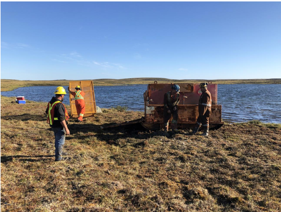
Figure 6. Fuel tank being extracted from the lake
