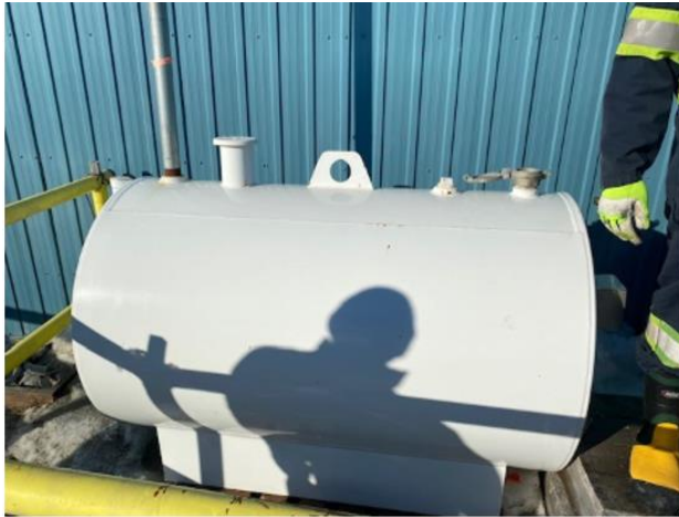
Figure 2: The exterior fuel tank and damaged fuel line which led to the spill.
