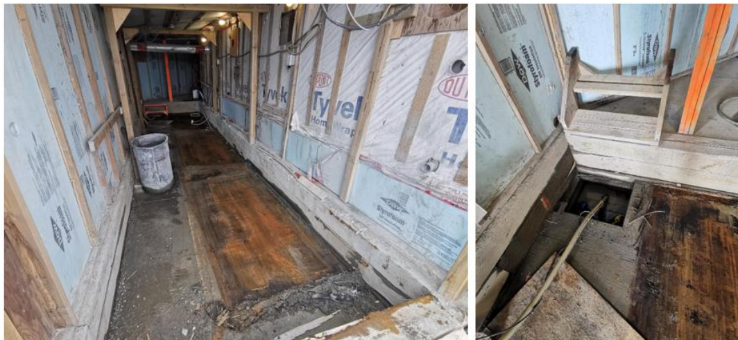
Figure 5: Decantation room cleared of all materials, and the down slope sump actively being pumped of standing diesel.
