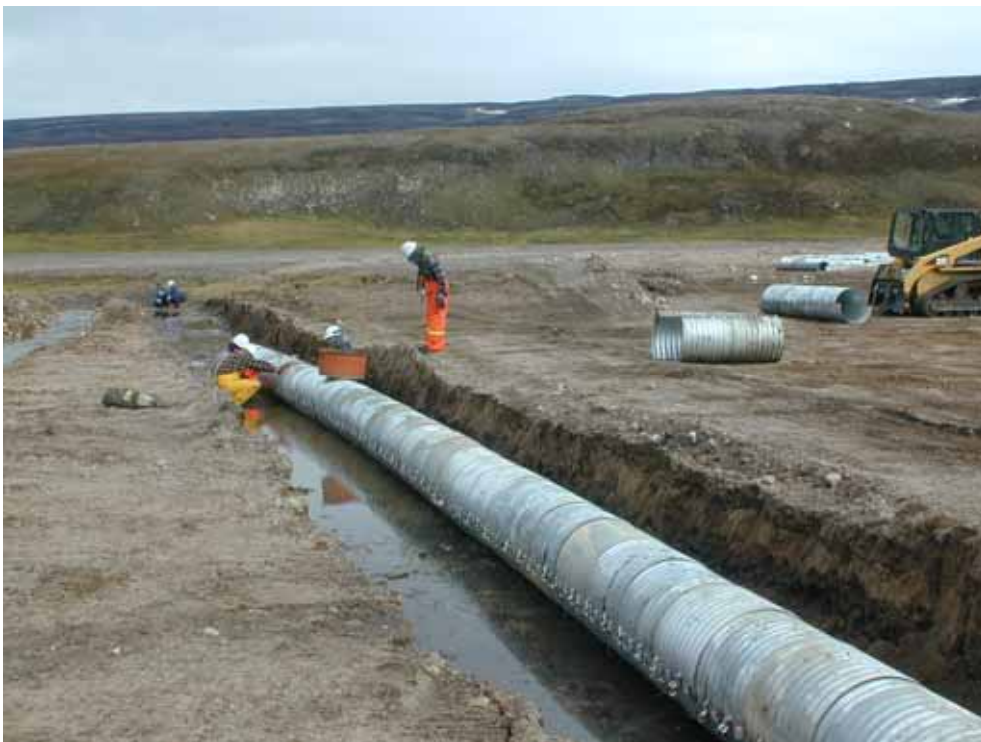
Use of Culvert Material to replace old 45-gallon drums and rehabilitate Mary River Airstrip. Material helped existing natural drainage and did not change any water-way.
