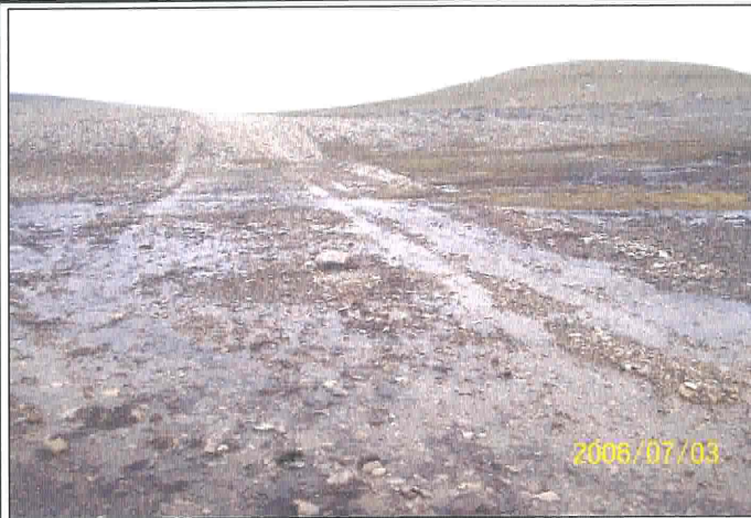
Looking north from ground (July 03, 2006).
