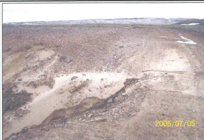
Looking north from ground (July 05, 2006).
