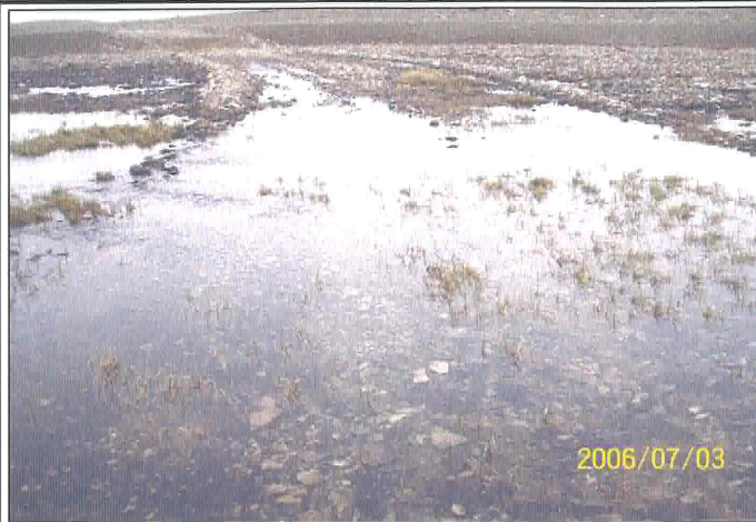
Looking north from ground (July 03, 2006).
