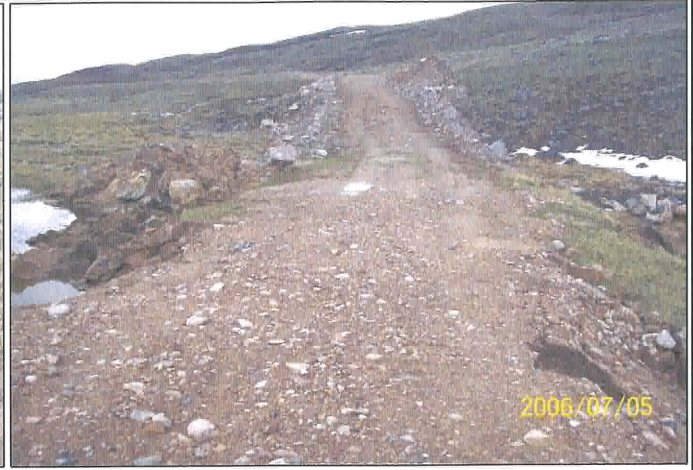
Looking north from ground (July 05, 2006).
