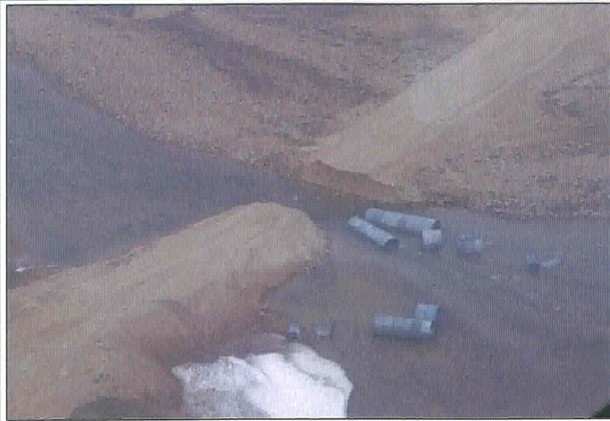
Looking south west from air (June 28, 2006).
