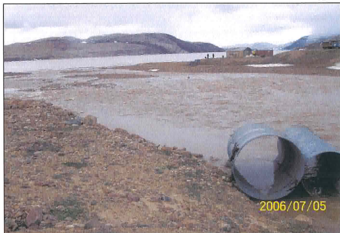
Looking north from ground (July 05, 2006).
