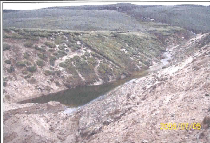
Looking north east from ground (July 05, 2006).
