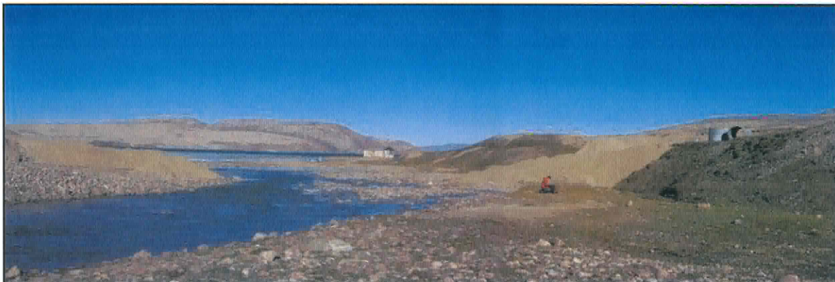
Panoramic View of Road Crossing - looking downstream
