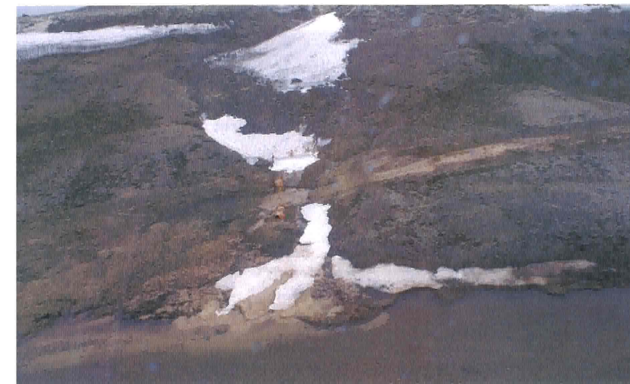
Photo 3 A washed out barrel culvert bypassed by a new channel.
