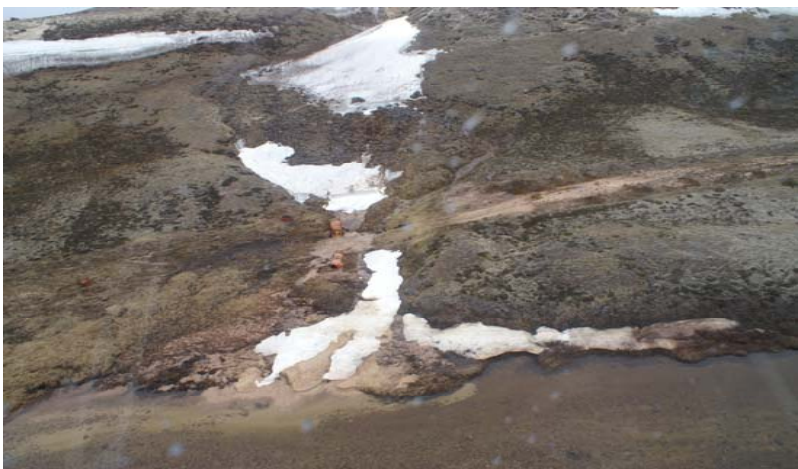
Photo 3: A washed out barrel culvert with a new channel.
