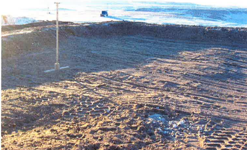
Photo 9: Appropriate amount of cover is being placed over the liner.
