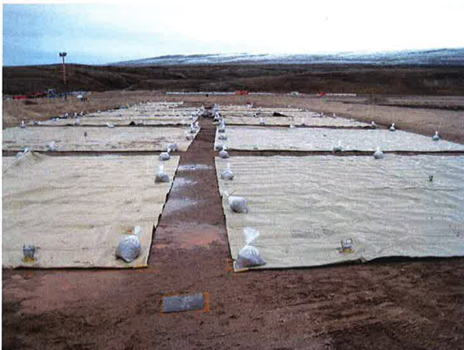
Photo 11: Fuel bladders are placed at their appropriate locations as per the design.
