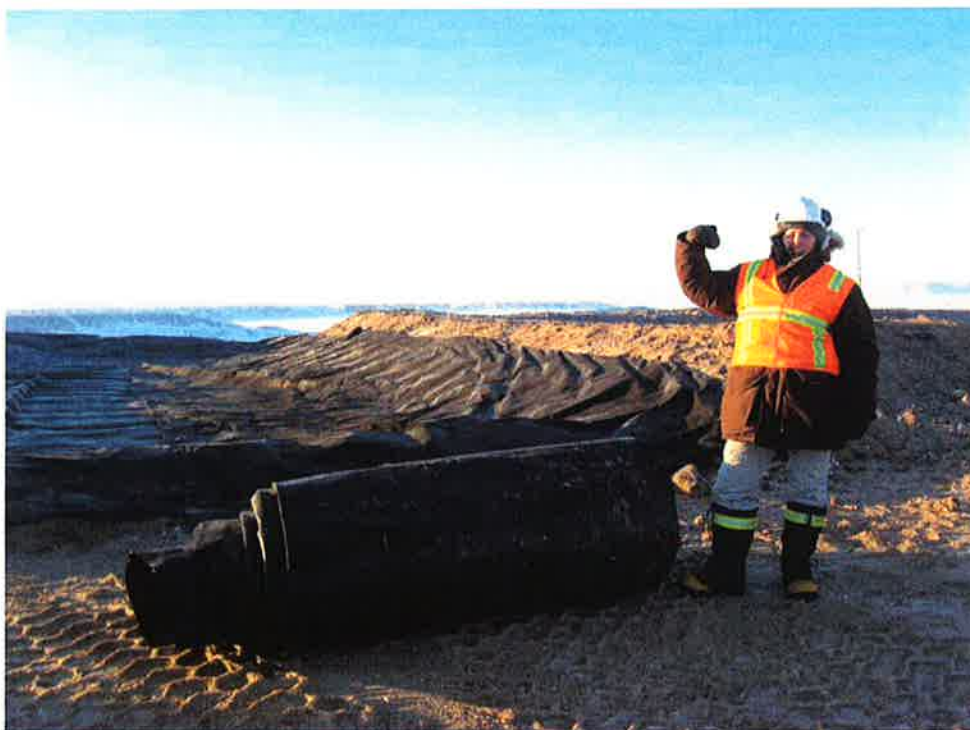
Photo 6: The liner is being installed within the containment and slopes.
