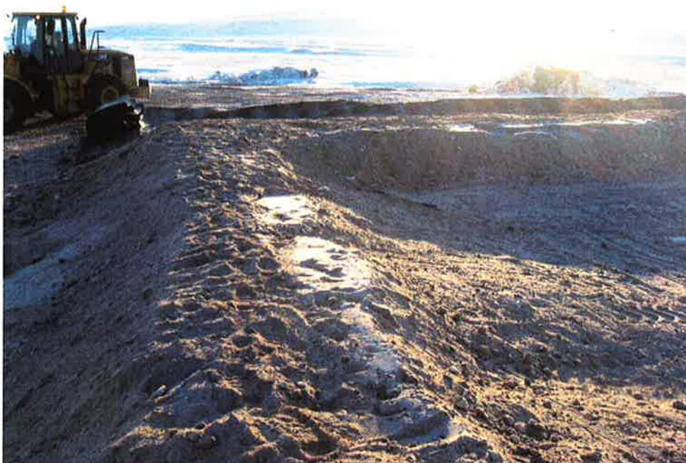
Photo 4: The slopes and the base are ready for the installation of the liner.
