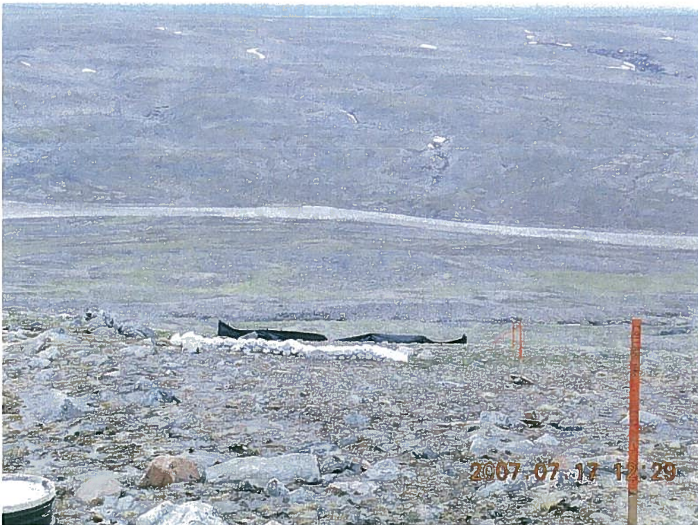
Photo 20: Silt fences (SF 5+6) and berms (B 1+2) at MR3-07-116 and MR3-07-120
