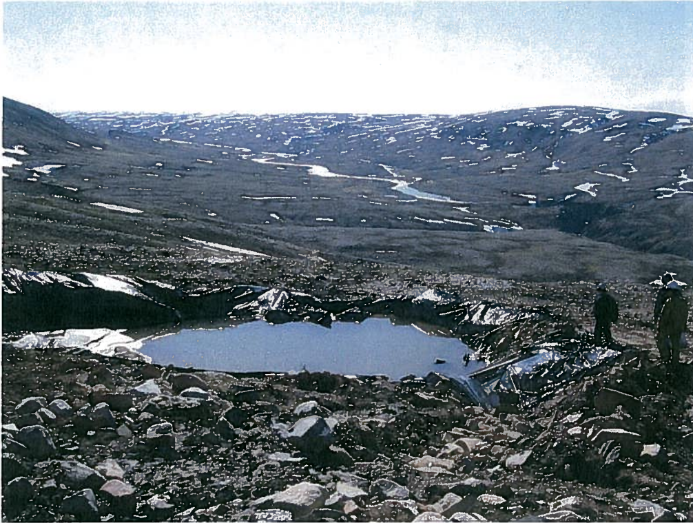
Photo 11: Axial sump (SU 6) with liner (photo 1)
