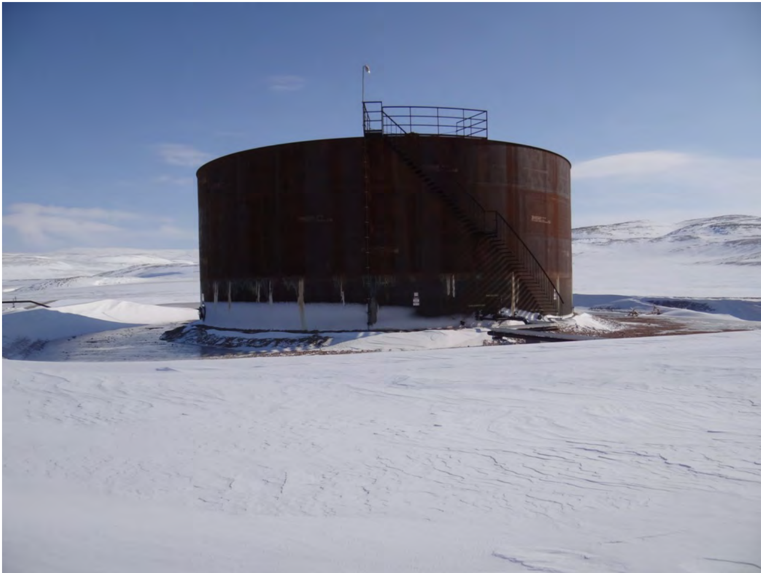
Single new 5M liter tank containing fuel at time of inspection- Milne Inlet
