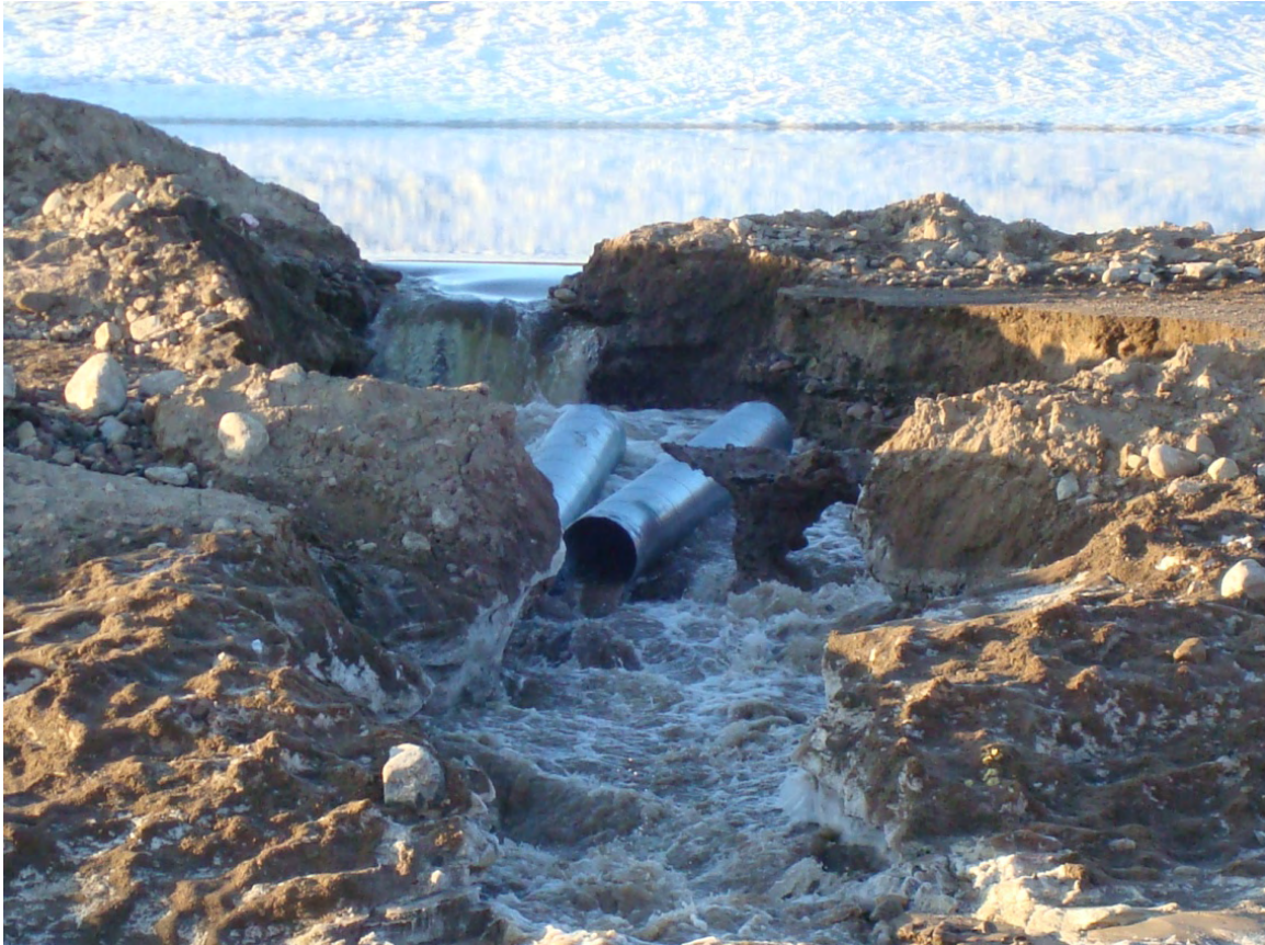
Photo 1: May 15, approximately 9 PM - View upstream showing washed out area of road and upstream pond.
