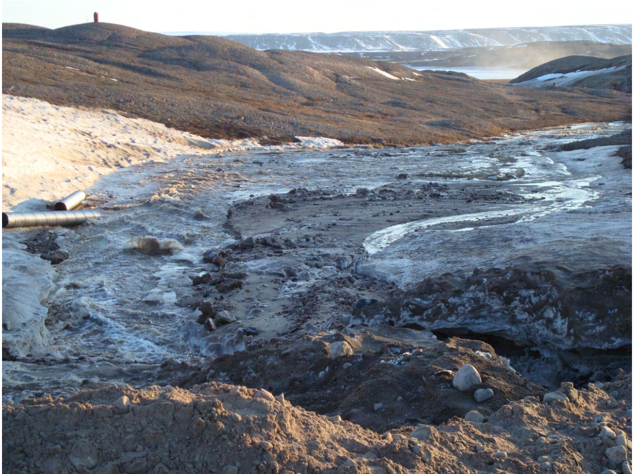
Photo 2: May 15, approximately 9:00 PM – View downstream showing high flows resulting from road wash, flows subsided within 2 hrs. Note two temporary culverts that were washed downstream during attempt to mitigate.
