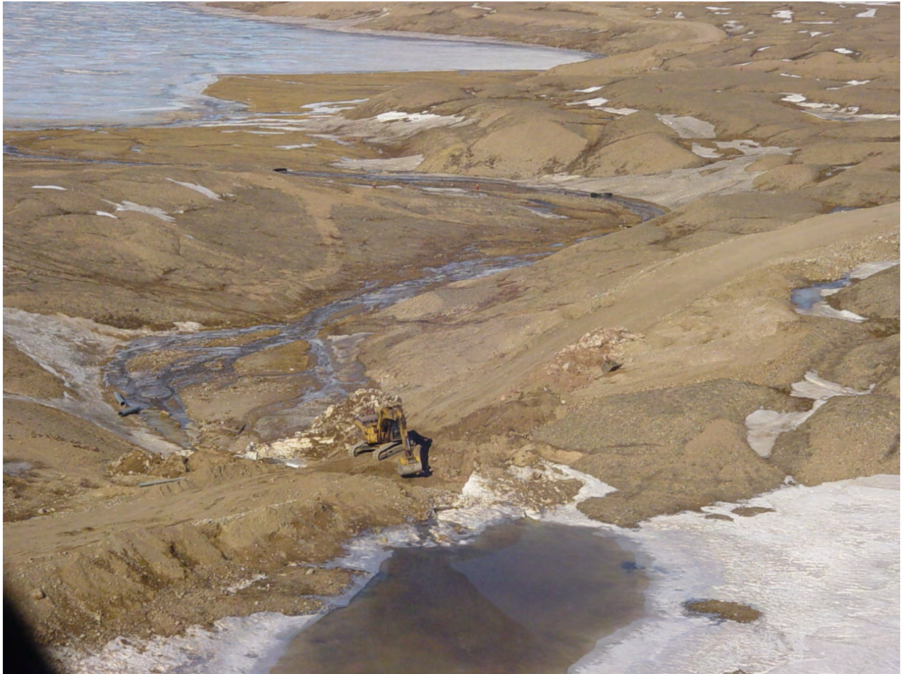
Photo 7: May 16, approximately 11 AM - Aerial view downstream from remnant of upstream pond, showing installation of auxiliary culvert.
