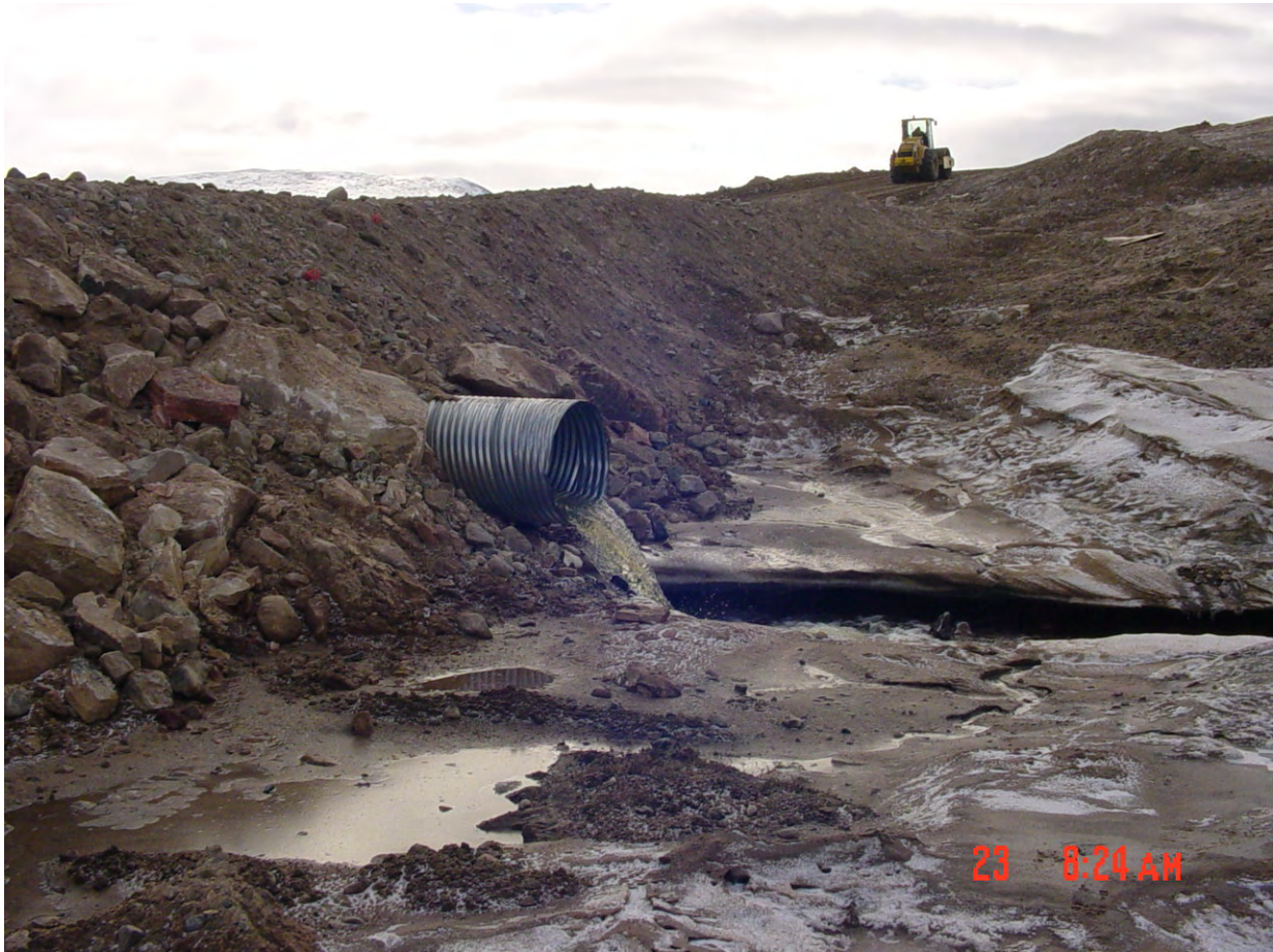
Photo 8: May 23 stream walk over - Perched downstream 'auxiliary' culvert. Original installed culvert is below, and not currently visible or open.
