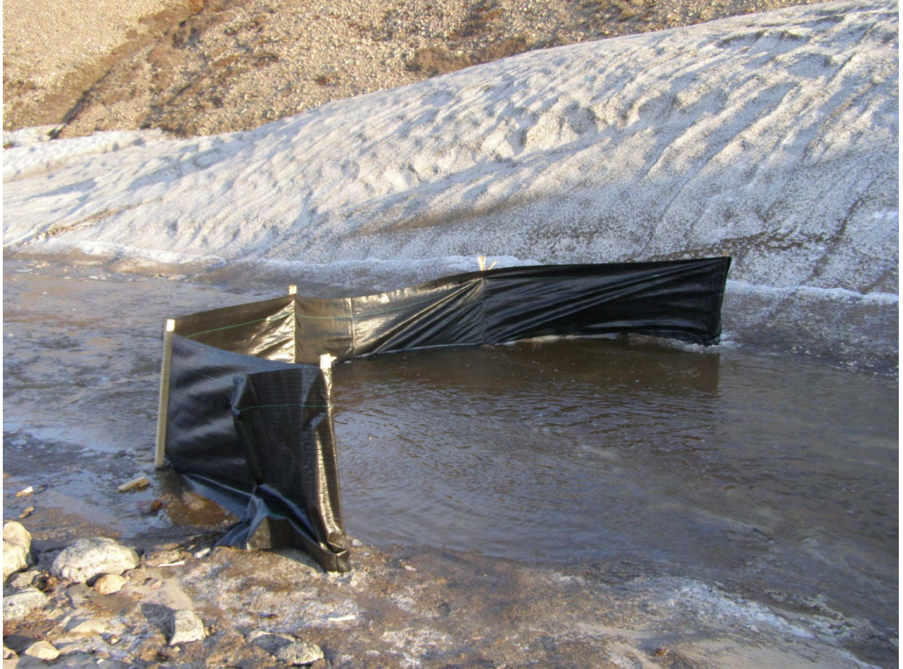
Photo 3: May 16 approximately 2 AM – View downstream - close-up silt fence installation
